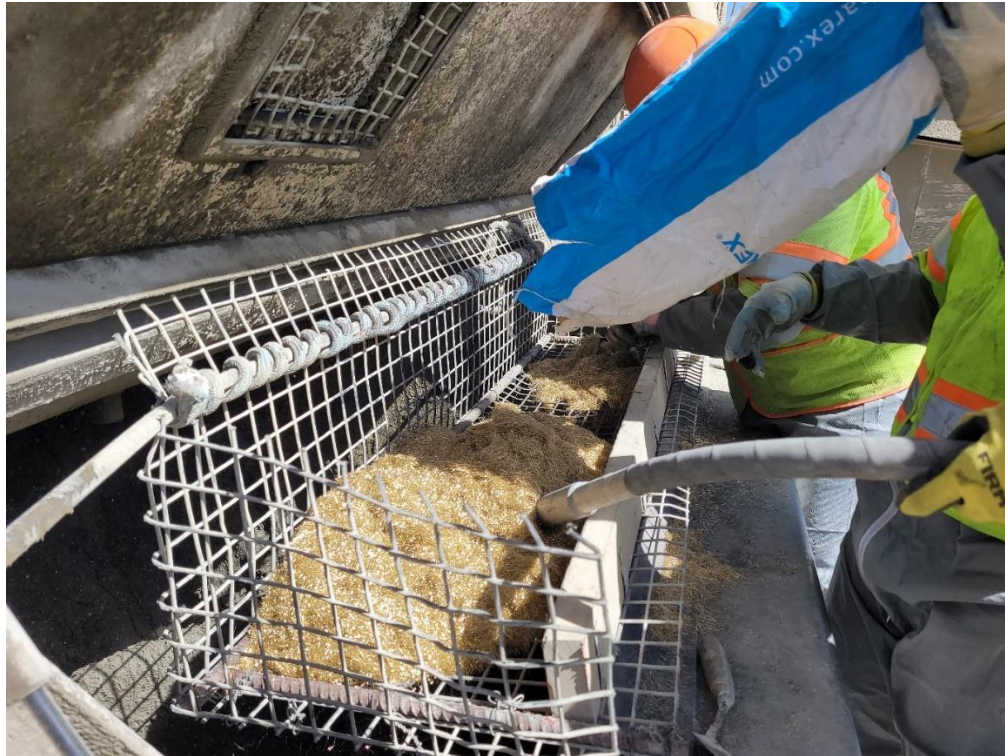
Figure 2.4. Screen and Vibrator used for Fiber Addition.
