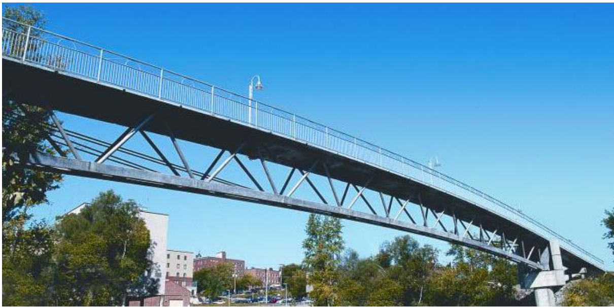
Figure 2.14. Sherbrooke Footbridge, Canada (Russell et al. 2013).
