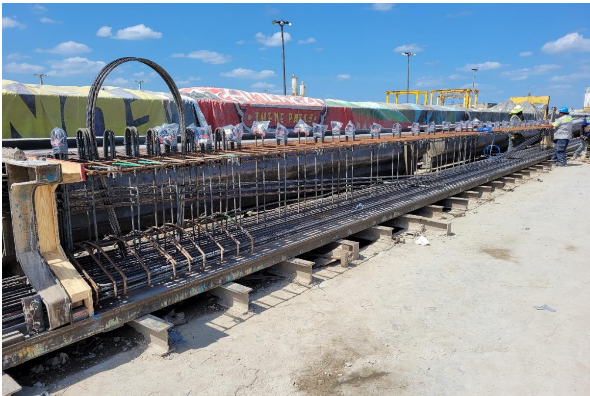
Figure 6.13. Tx34-2 Prestressing and Reinforcement on the Casting Bed.
