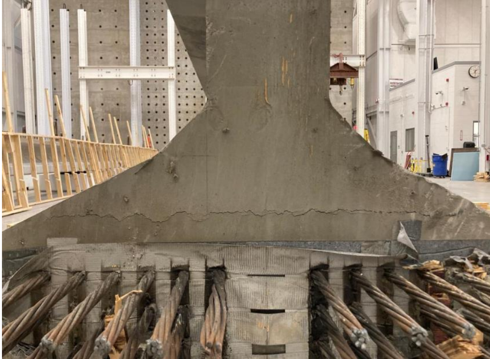
(a) Lower Transition Line at East End
