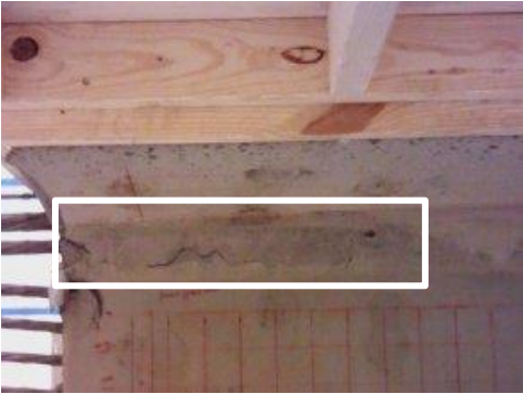
(c) FLIR Digital Image—South-west
