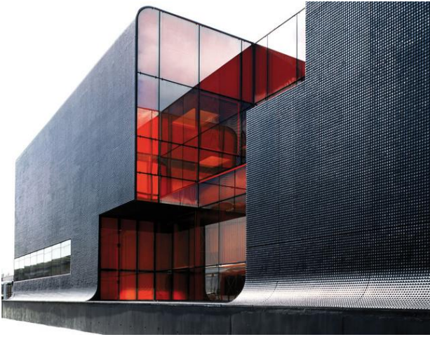
(a) RATP Bus Center, France (Batoz and Behloul 2011)
