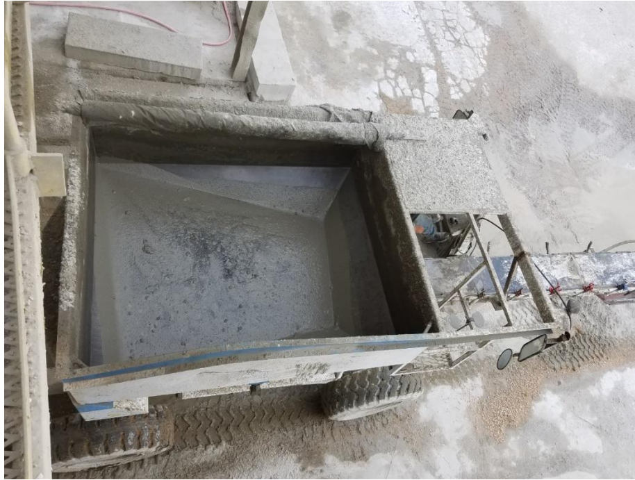
Figure 6.6. Fresh UHPC Discharged into a Tuckerbuilt Concrete Transporter.
