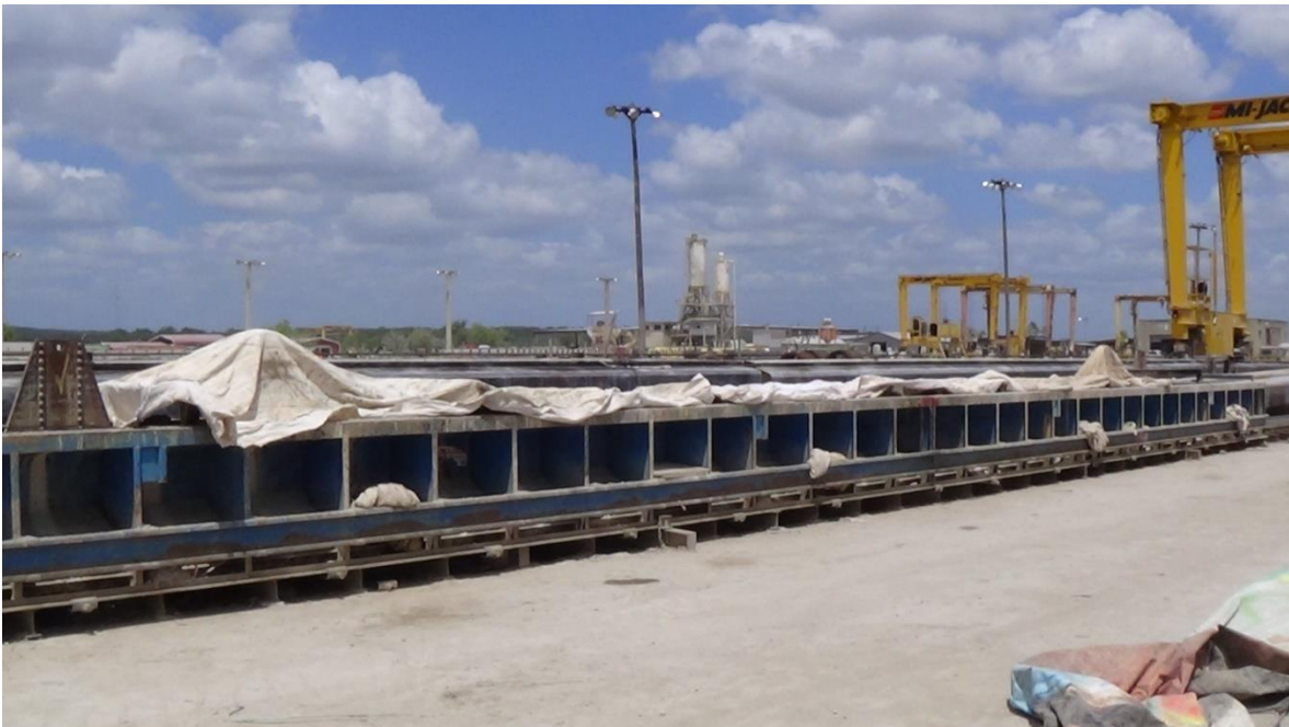
Figure 6.15. UHPC Covered after Casting.
