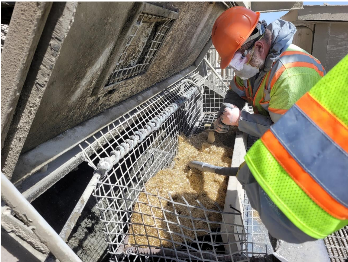
Figure 6.21. Manual Addition of Steel Fibers for Tx54.
