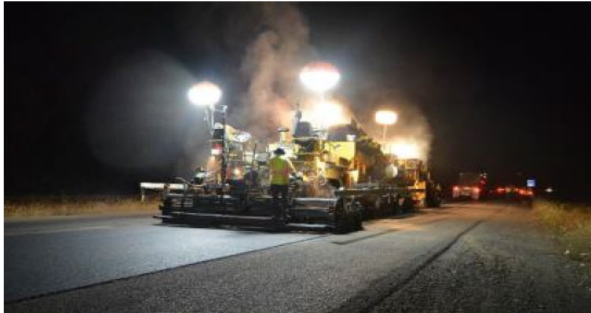
Figure 36. Balloon Lights Mounted on Paver (Gambatese, J., And Jafarnejad, A.,2018).
