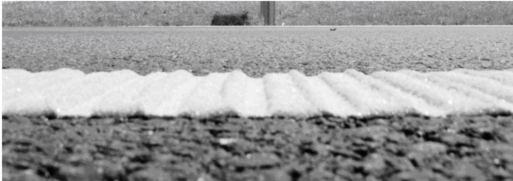
Figure 54. Typical inverted-profile thermoplastic marking (Carlos, A., & Lopez, P., 2004)
