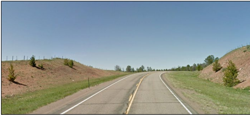
Figure 7: Section of Happy Jack Road with restricting sight distance.
