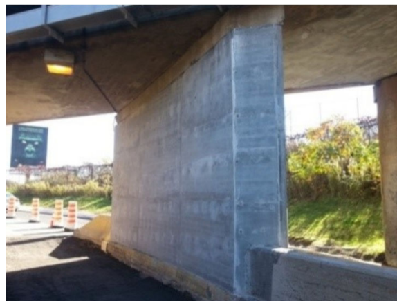
Figure 2.29 Finished Surface ( Doiron 2016 )
