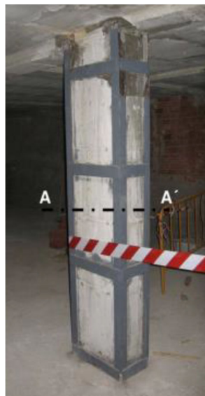
Figure 2.3 Completed Steel Jacketing (Islam & Hoque 2017, p. 7)
