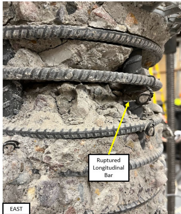
Figure 3.50 Precast 1 Ruptured Longitudinal Bar, East Face
