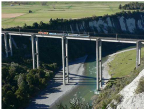
(a) South Rangitikei Viaduct
