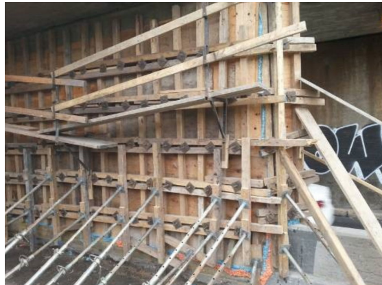
Figure 2.28 Setting-up the Formwork for Casting ( Doiron 2016 )
