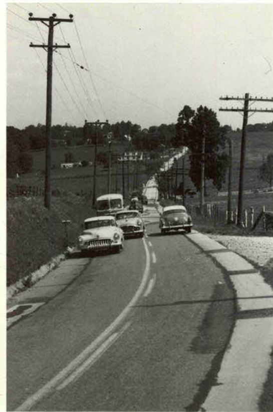
By the 1950's, most early unsurfaced rural roads had been paved and widened. Nevertheless, many of these roads were still dangerously narrow, resembling this one photographed in 1953.
