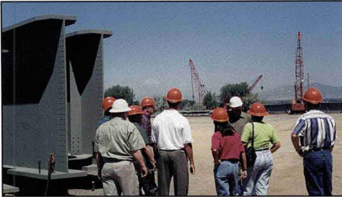
Engineers frequently visit job sites to monitor construction progress. Here a group is inspecting some of the girders that will make up part of a bridge on the I-15 project in Salt Lake City, UT.
