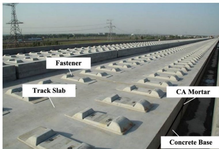
Figure 2-12. Photo of ballastless track system [39].
