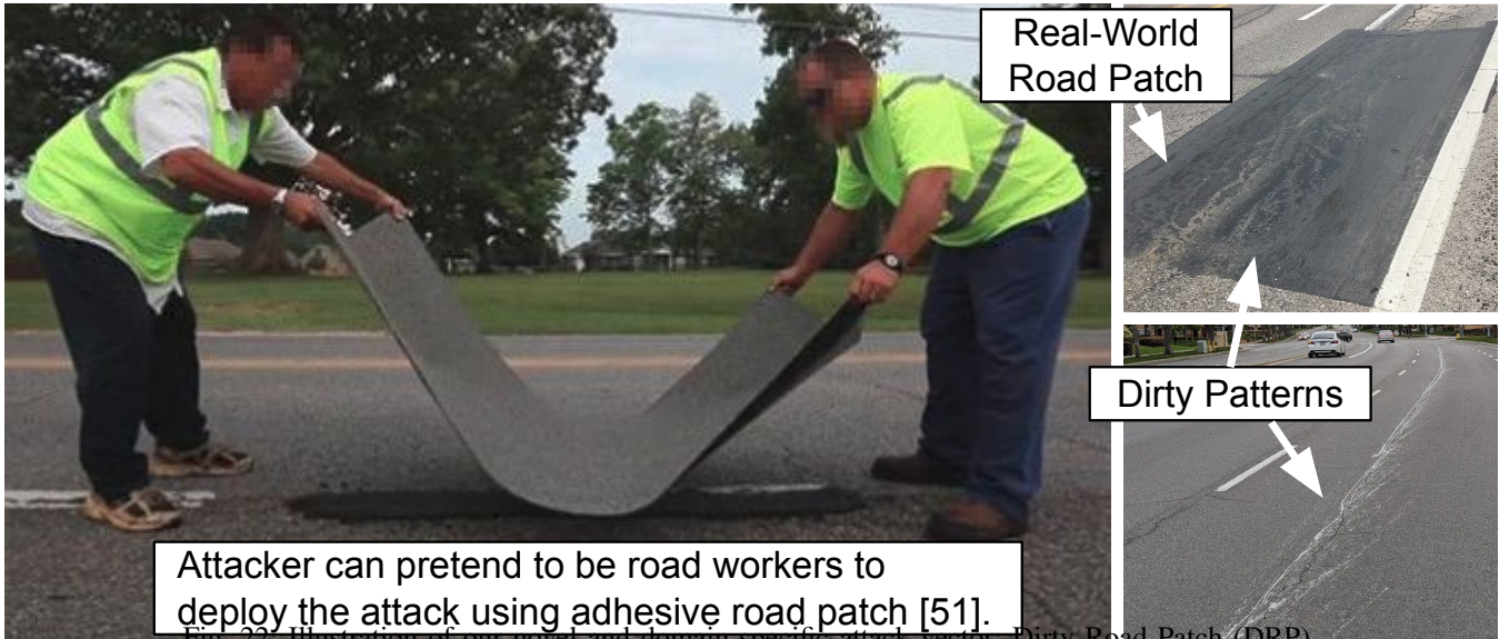
Fig. 22. Illustration of our novel and domain-specific attack vector, Dirty Road Patch (DRP).
