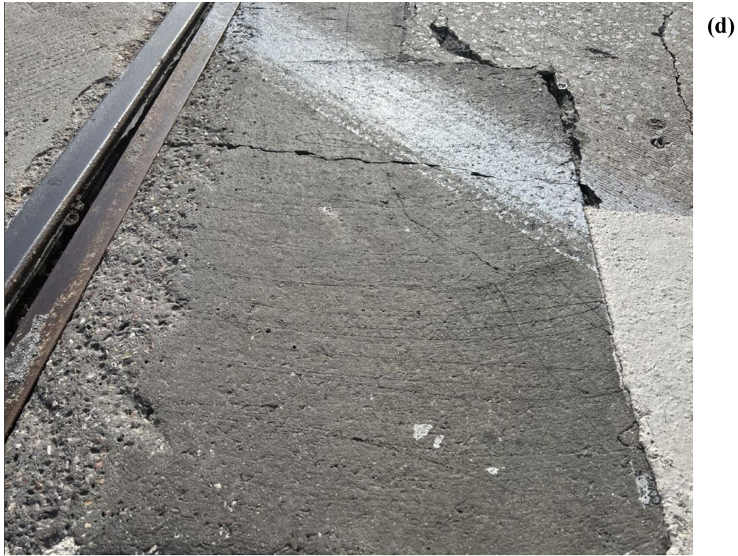
Figure A.3 (continued) Current state of repair material installed at location 3
