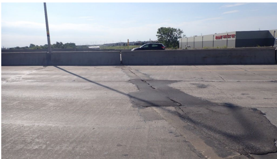
Figure A.10 (continued) Current state of repair material installed at location 3
