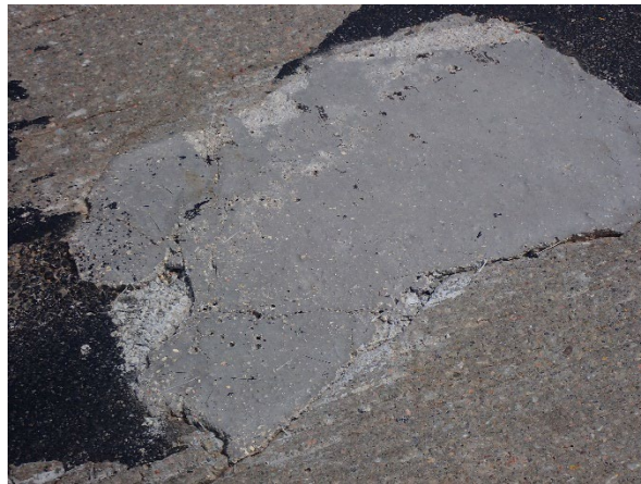
Figure A.18 (continued) Current state of repair materials installed at location 2
