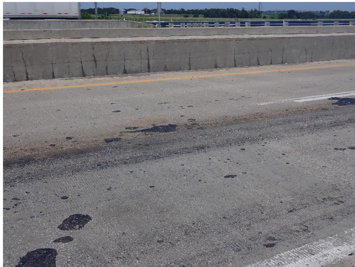
Figure A.23 (continued) Current state of repair material installed at location 7
