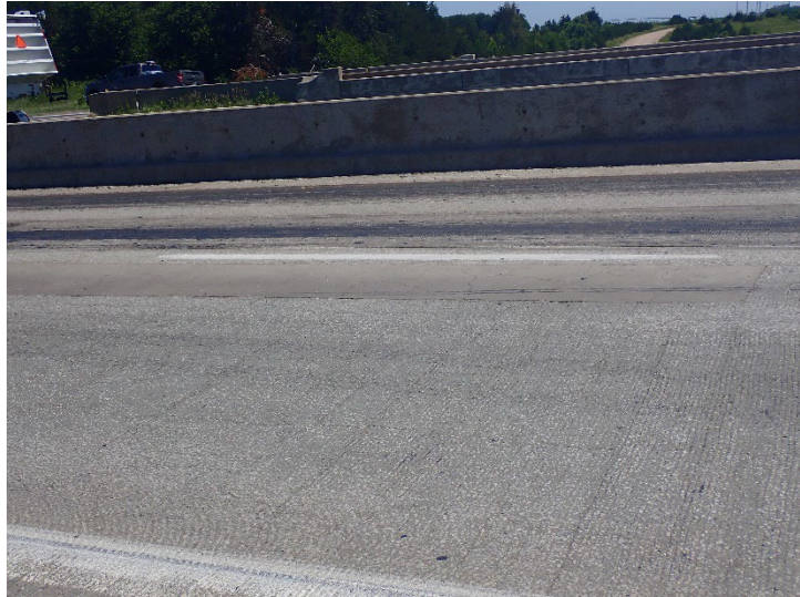
Figure A.22 (continued) Current state of the repair material used in location 6
