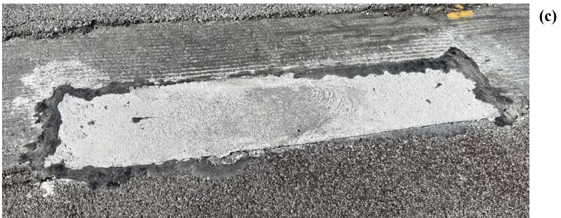
Figure Appendix A.7 Current state of repair material installed at location 7
