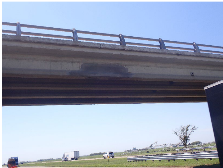
Figure Appendix A.24 Current state of repair material installed at location 8
