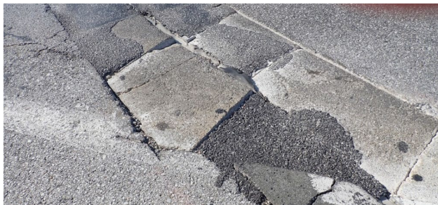
Figure A.8 (continued) Current state of repair material installed in location 1
