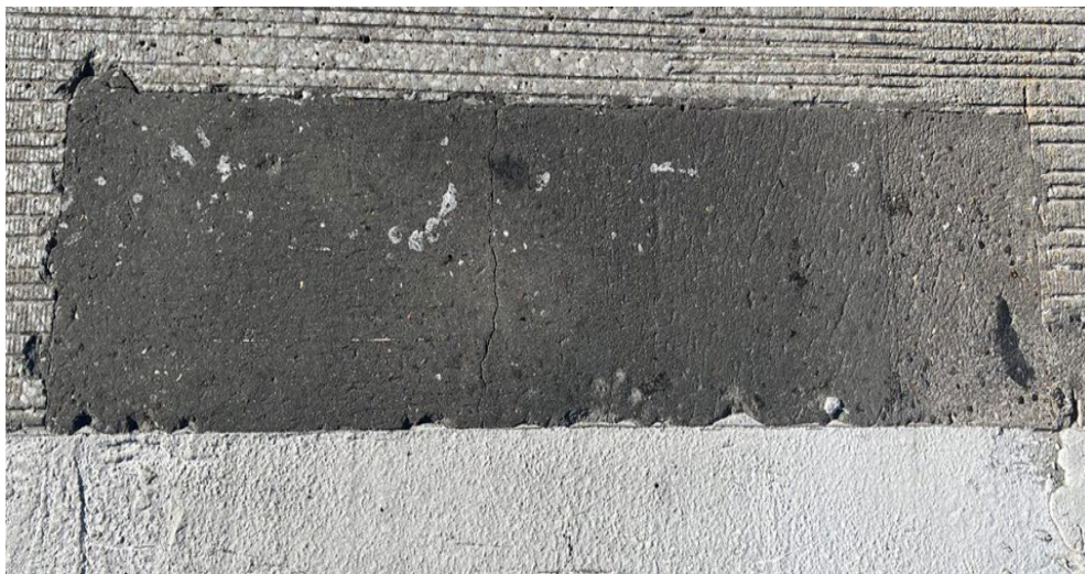
Figure Appendix A.1 Current state of repair material installed in location 1
