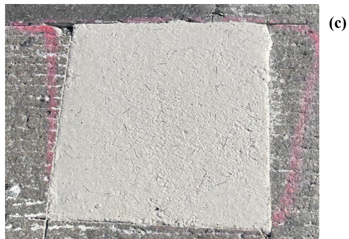
Figure Appendix A.5 Current state of repair material installed at location 5
