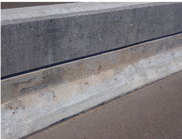
Figure Appendix A.19 Current state of repair materials installed at location 3
