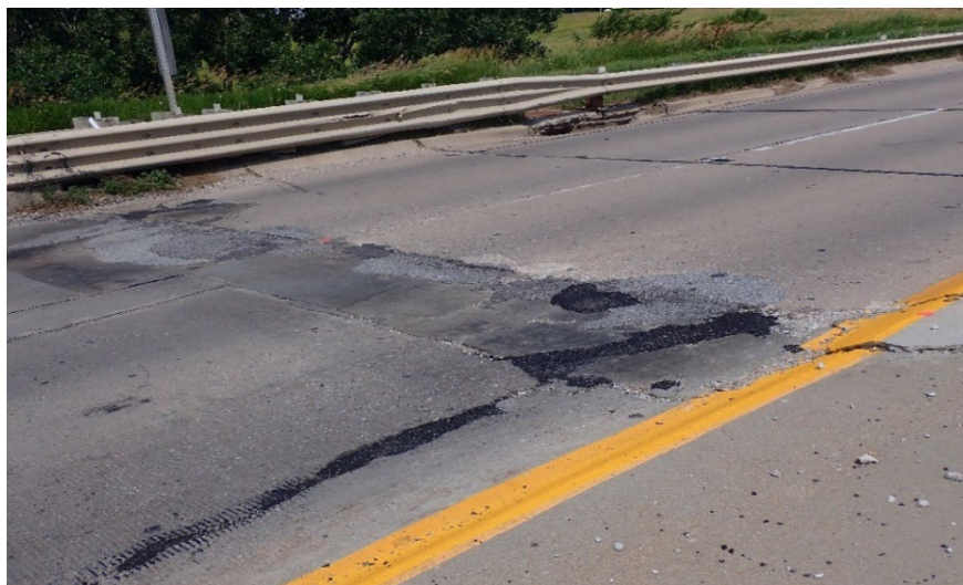
Figure Appendix A.16 Current state of repair material installed at location 9
