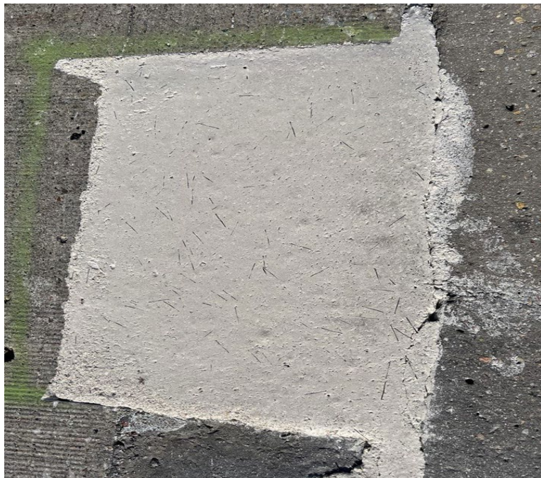
Figure A.4 (continued) Current state of repair material installed at location 4
