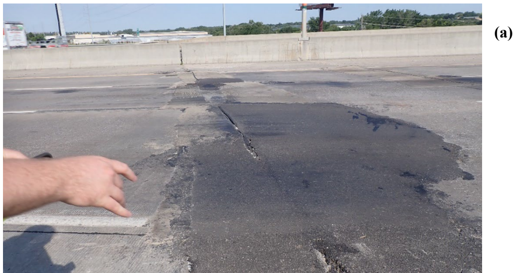
Figure Appendix A.12 Current state of repair material installed at location 5
