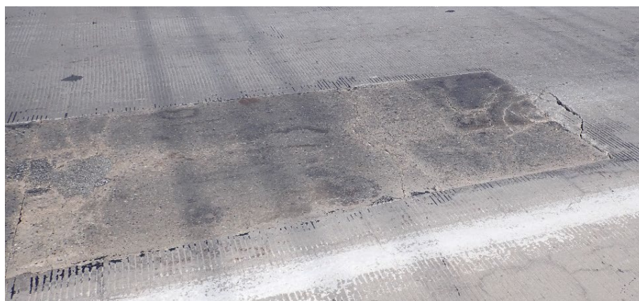
Figure Appendix A.13 Current state of repair material installed at location 6
