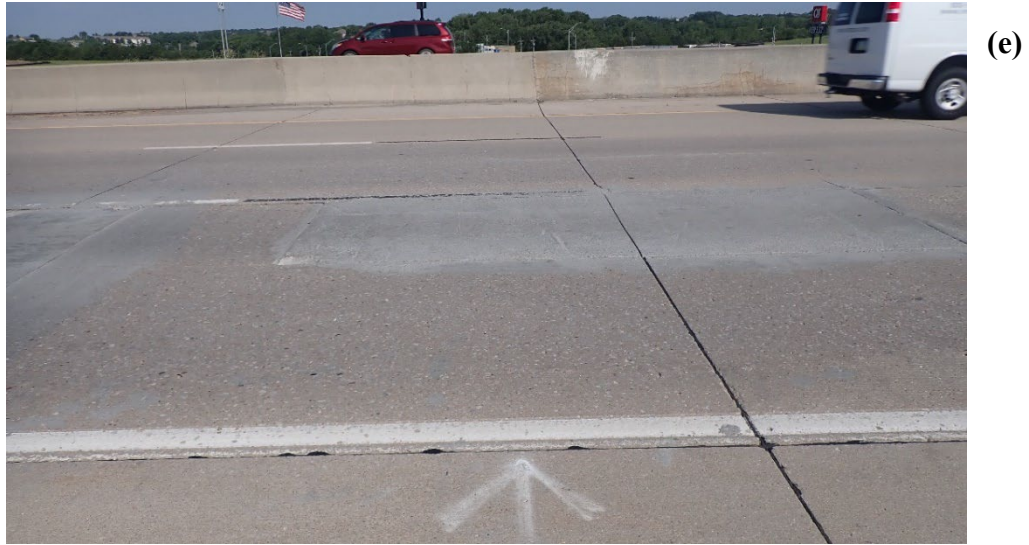
Figure A.11 (continued) Current state of repair material installed at location 4
