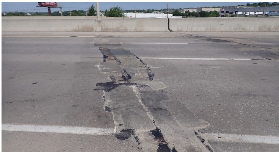
Figure A.12 (continued) Current state of repair material installed at location 5
