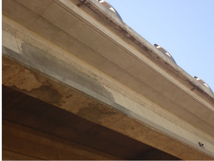
Figure A24 (continued) Current state of the repair material used in location 8
