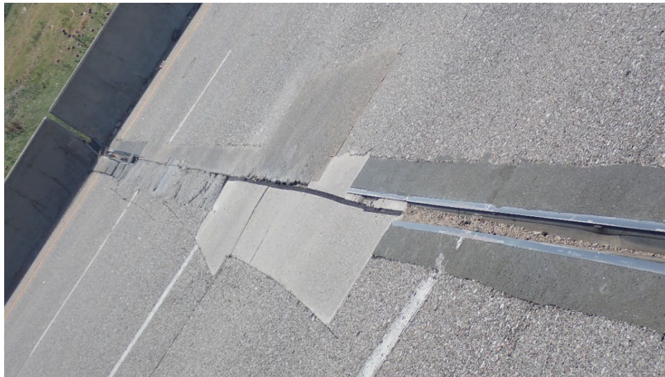
Figure A.14 (continued) Current state of repair material installed at location 7
