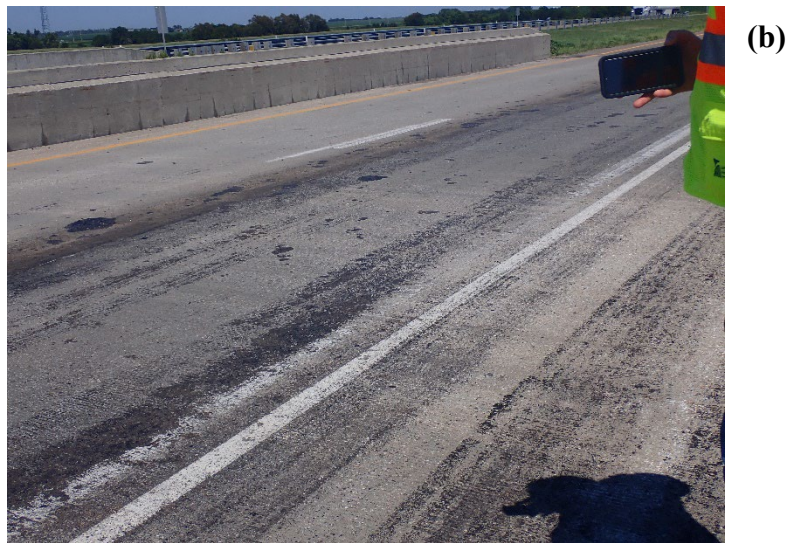
Figure Appendix A.23 Current state of repair material installed at location 7
