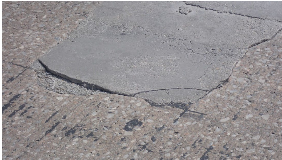
Figure A.15 (continued) Current state of repair material installed at location 8
