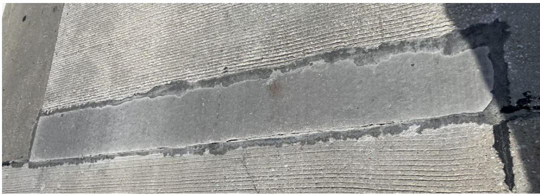
Figure Appendix A.6 Current state of repair material installed at location 6
