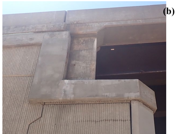
Figure Appendix A.20 Current state of the repair material used in location 4
