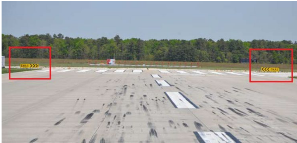
Figure 4. Location of EMAS Information Signs at the End of Runway 4 at ACY Airport
