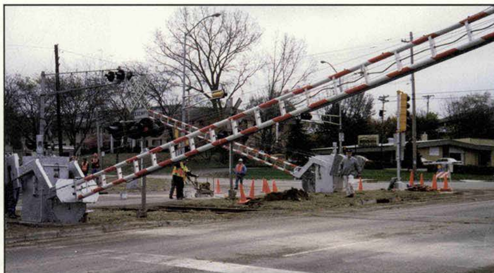
Safety barrier gates, like this system installed in Madison, WI, are designed to halt a pickup truck traveling at 40 mph.
