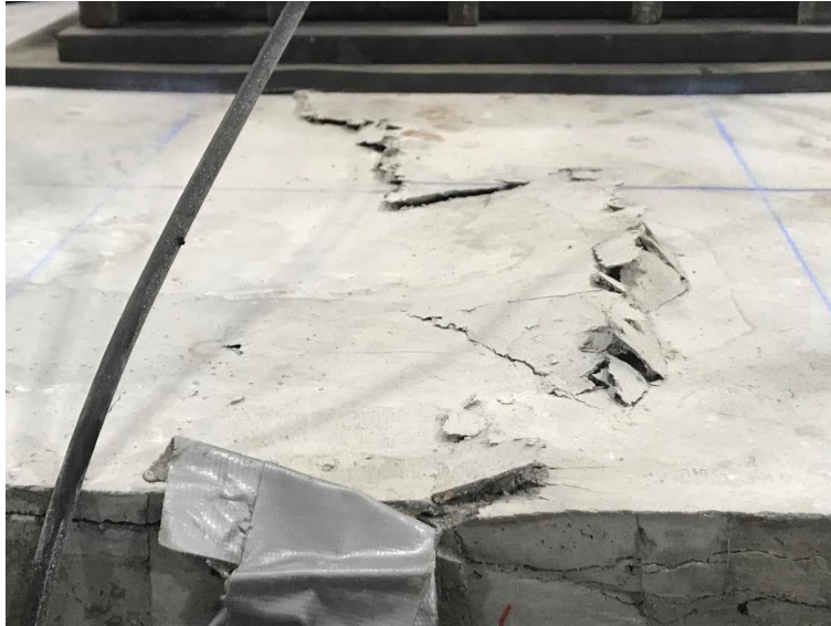
Figure 4.30. Crushing occurring at the midspan of the approach slab at failure, Test 2
