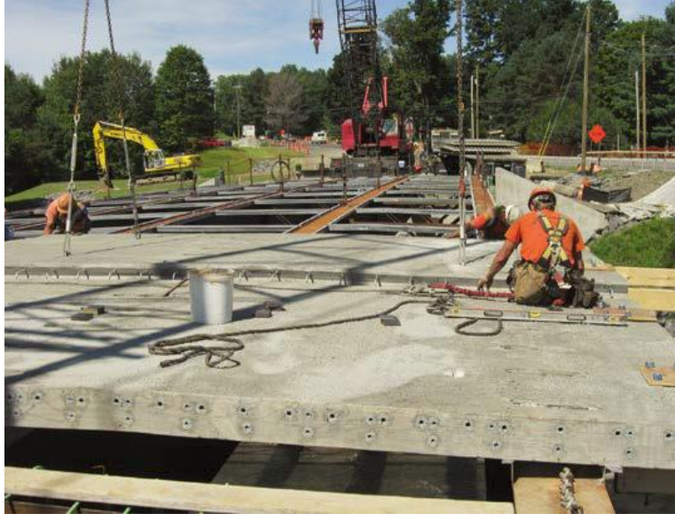
Royce 2016, NYSDOT Office of Structures
