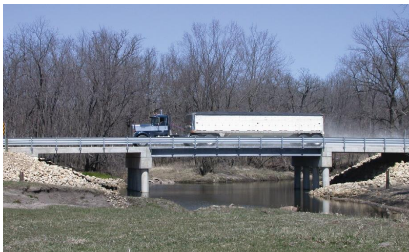
Bridge Engineering Center 2011
