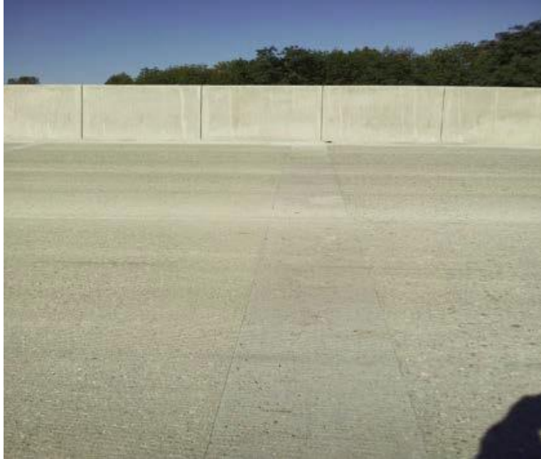
Figure 2.17. Finished NYSDOT link slab
