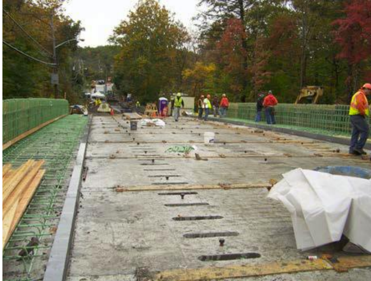
Royce 2016, NYSDOT Office of Structures
