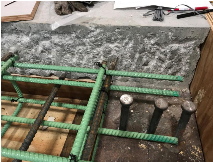
Figure 4.4. Jack hammering performed on construction joint to increase bond strength
