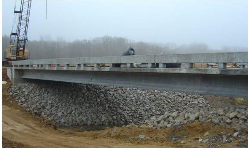
Bridge Engineering Center 2008
