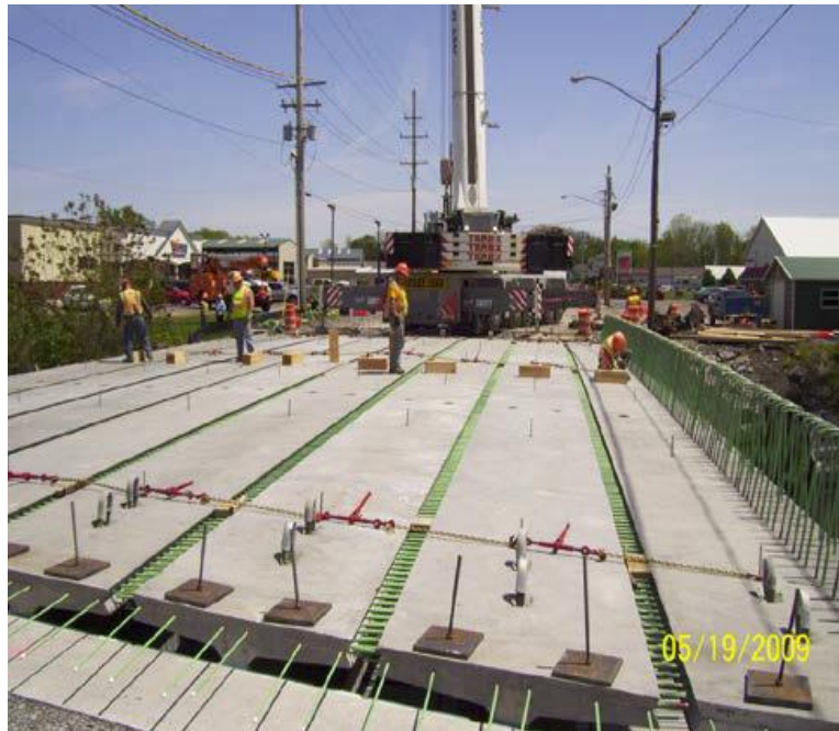
Royce 2016, NYSDOT Office of Structures
