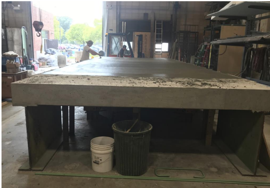
Figure 4.2. Laboratory specimen after concrete for approach slab and diaphragm sections was placed, with steel girders visible
