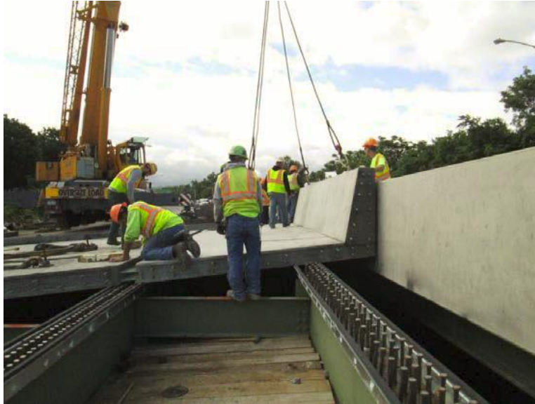
Royce 2016, NYSDOT Office of Structures
