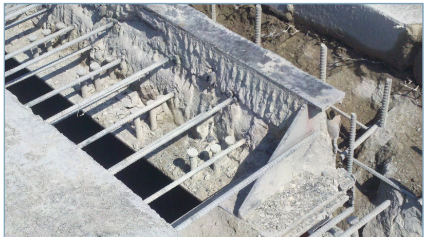
Sliding plate joint anchorage observed during removal in the first phase of the research project
