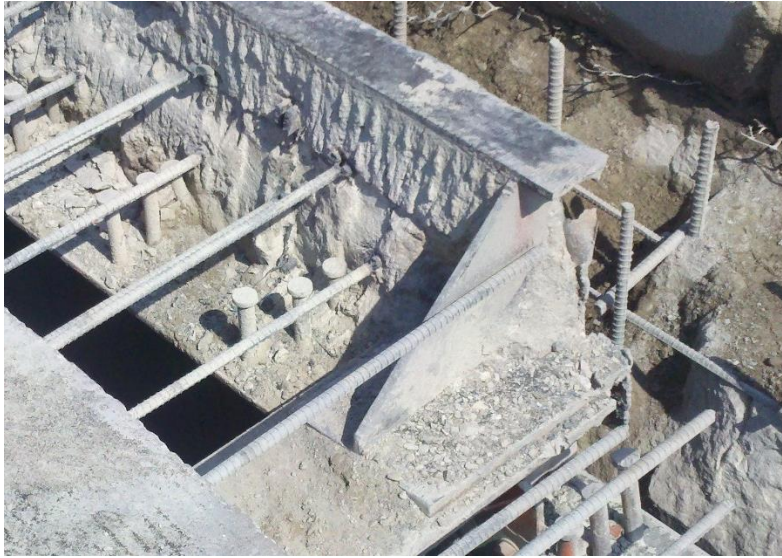
Figure 6.8. Sliding plate joint anchorage during removal
