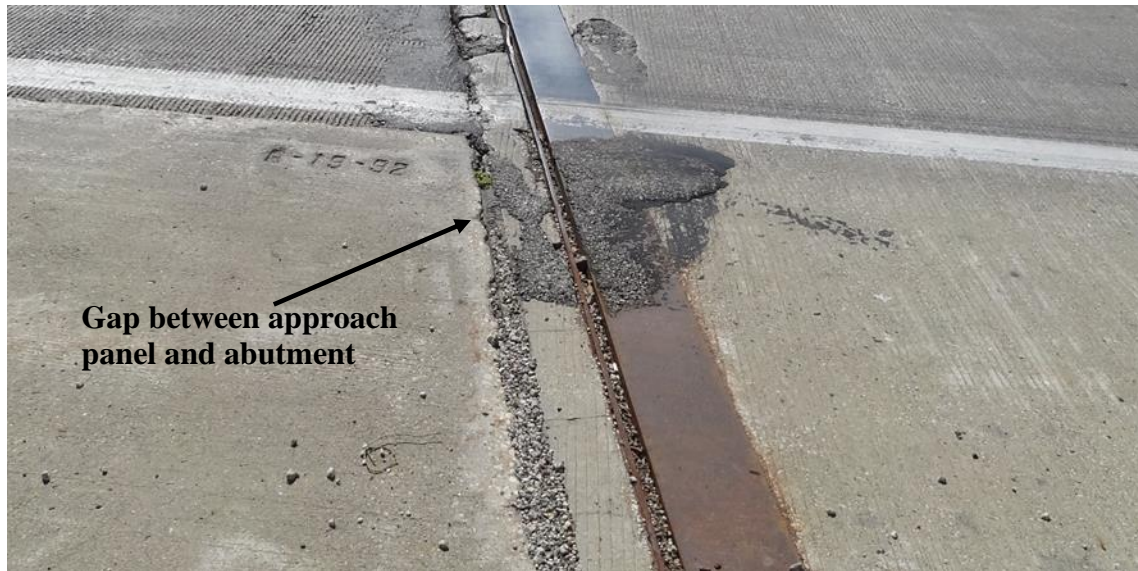
Figure 3.2. Gap forming between top of abutment and approach panel on the I-80 over I-35 west abutment in Iowa
