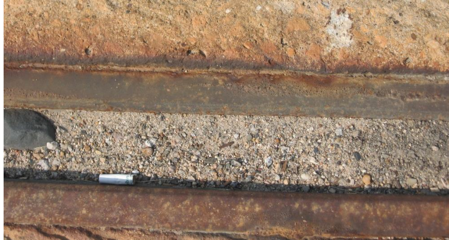
Figure 3.7. Badly weathered, but still functioning, strip seal joint showing debris building up in the seal
