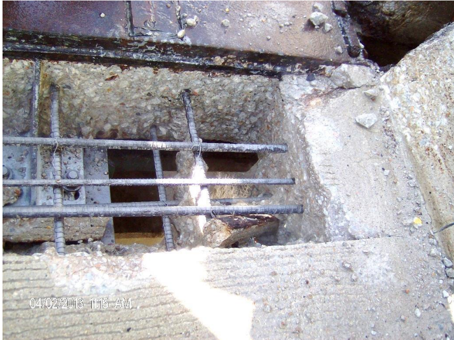
Figure 4.6 Concrete remaining after hydrodemolition
