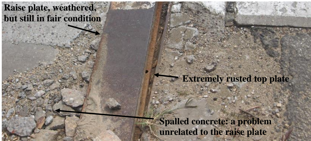
Figure 3.3. Rusted top plate beneath a raise plate showing relatively good condition on westbound US 20 over Catfish Creek in Cedar Rapids, Iowa
