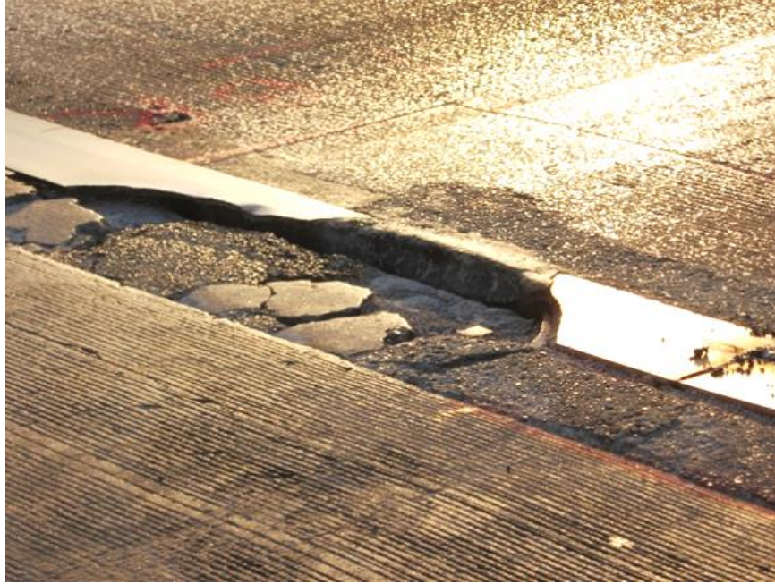
Figure 3.1. Large sections of a plate broken loose on northbound I-380 Exit 19A in Cedar Rapids, Iowa
