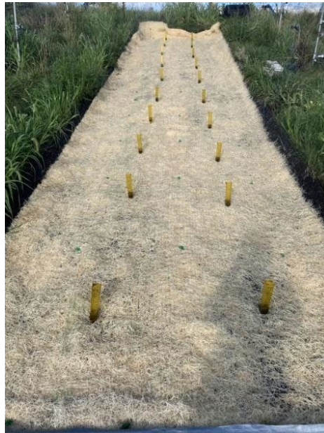
Figure 20. Photo. American Excelsior Curlex® II placed on the slope.
