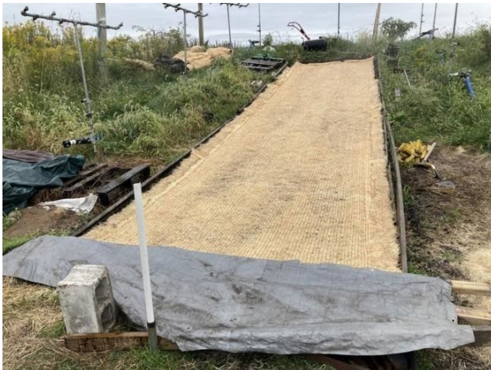
Figure 25. Photo. American Excelsior Curlex® II FibreNet placed on a slope.
