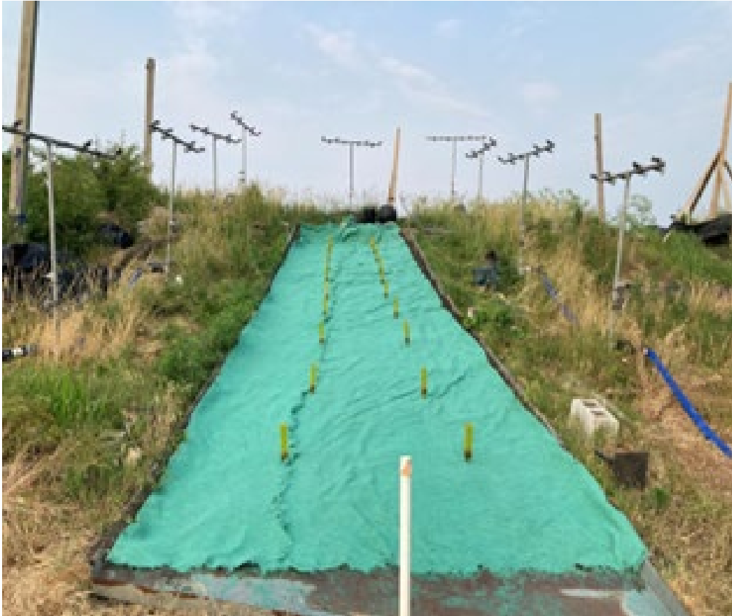
Figure 28. Photo. Profile F4 Netless placed on the slope.
