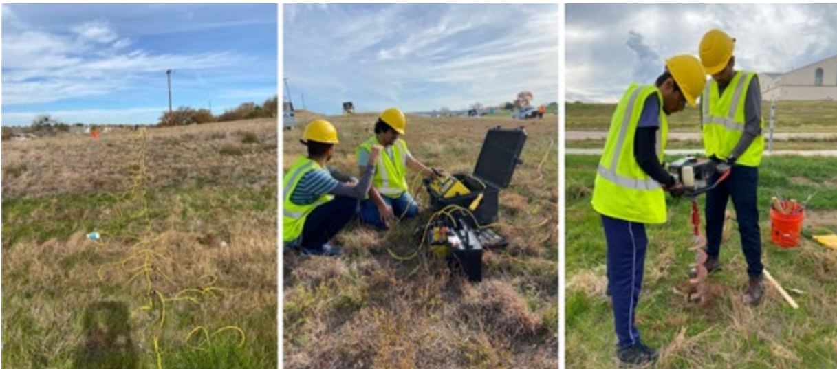
Figure 4.19. Implementation of ERI along Highway US 67 and soil sample collection
