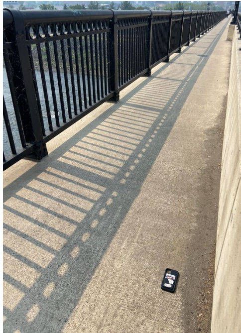
Figure 8 : Placement of smartphone on sidewalk for initial testing of Fahy Bridge.
