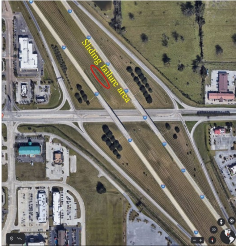
Figure 16. Aerial view of I-10 @ LA30 embankment site
