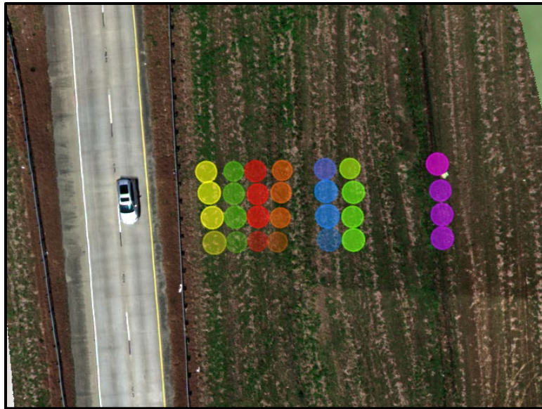
Figure 54. Orthomosaic map near the failure area for I-10 @ LA30 embankment
