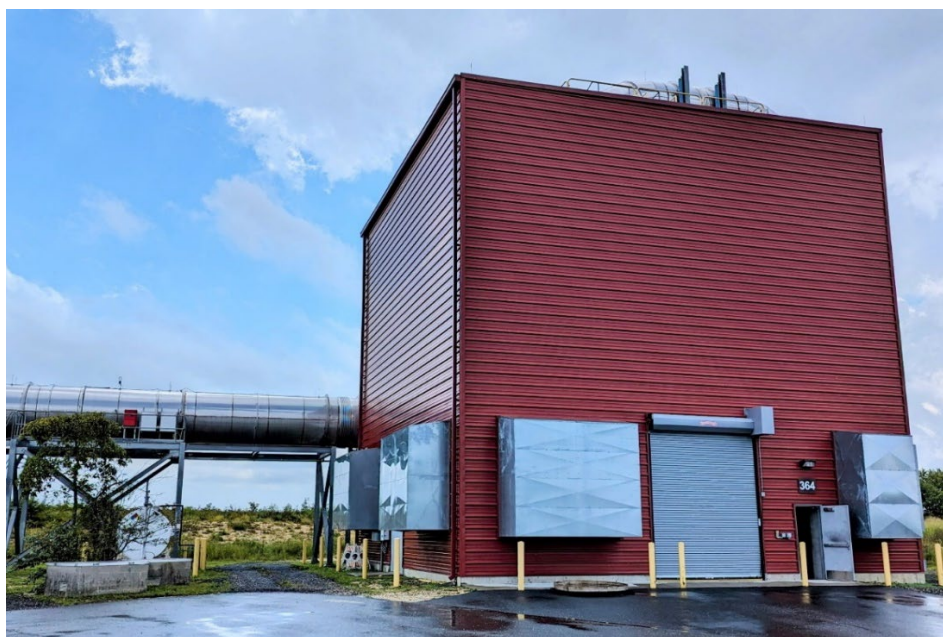
Figure 1. Exterior of Fire Test Facility
