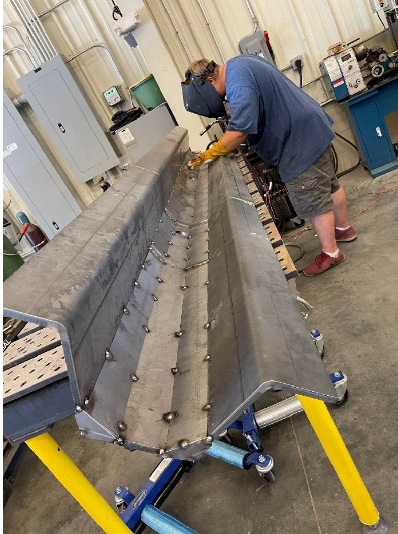
Figure 4.20 Welding of an outside cover for strain gauges.
