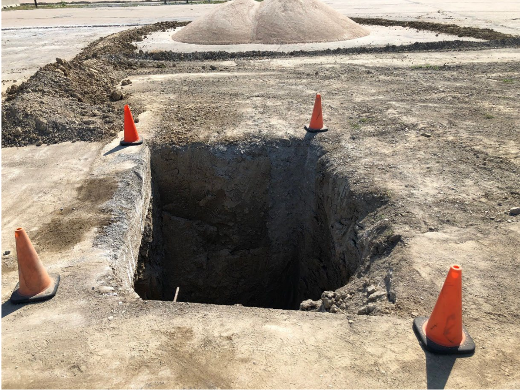
Figure 4.5 A photo of the test pit after excavation.
