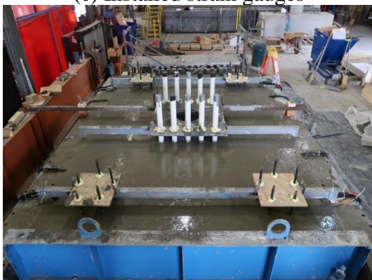
(e) Concrete placement
