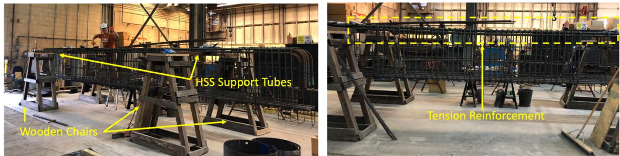
Figure 6-8 Fabrication setup for cage assembly
