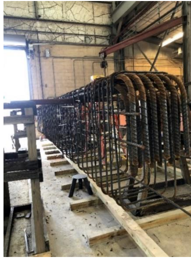
(b) Stirrups and web reinforcement
