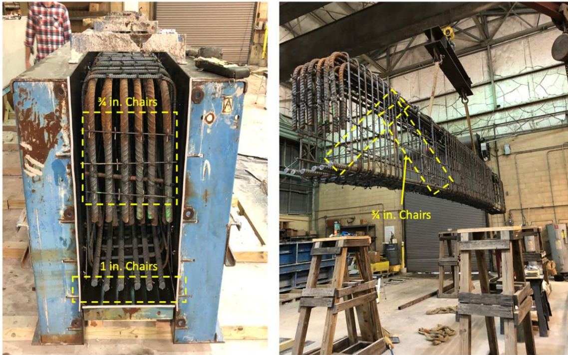
Figure 6-11 Cage lift onto steel soffit and placement in formwork
