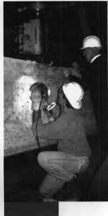
Researchers at FHWA's Turner-Fairbank Highway Research Center test a beam of high-performance concrete.
