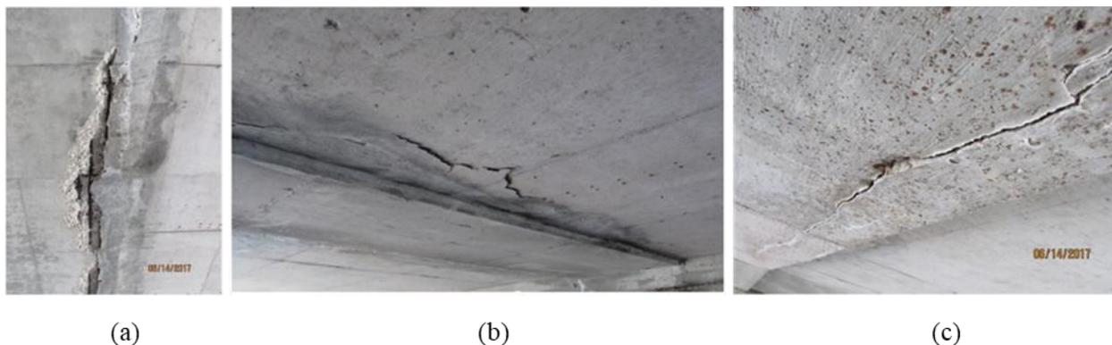
**Figure 2. 2 Deterioration observed in past studies: (a) spalled concrete, (b) delaminated area, and (c) large longitudinal crack in vicinity of longitudinal construction joint (Weatherer and Hedegaard 2019).**
