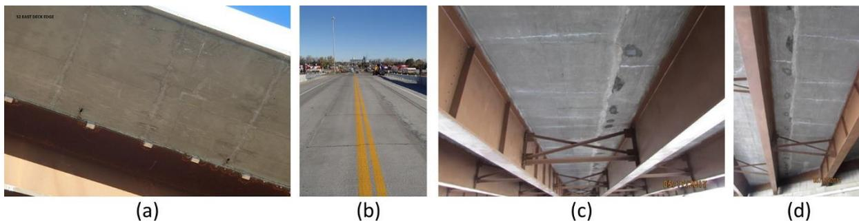
**Figure 1. 2 Evidence of cracking in second phase decks and/or closure pour regions: (a) and (b) S080-21180 2015 inspection (photos courtesy of NDOT); (c) and (d) from (Weatherer 2017).**
