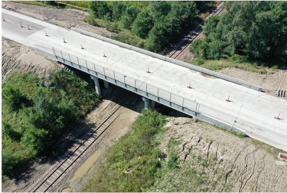
**Figure 4. 2 Aerial photo of the Brunswick Viaduct Bridge (Bridge 1) after deck replacement and prior to asphalt overlay**
