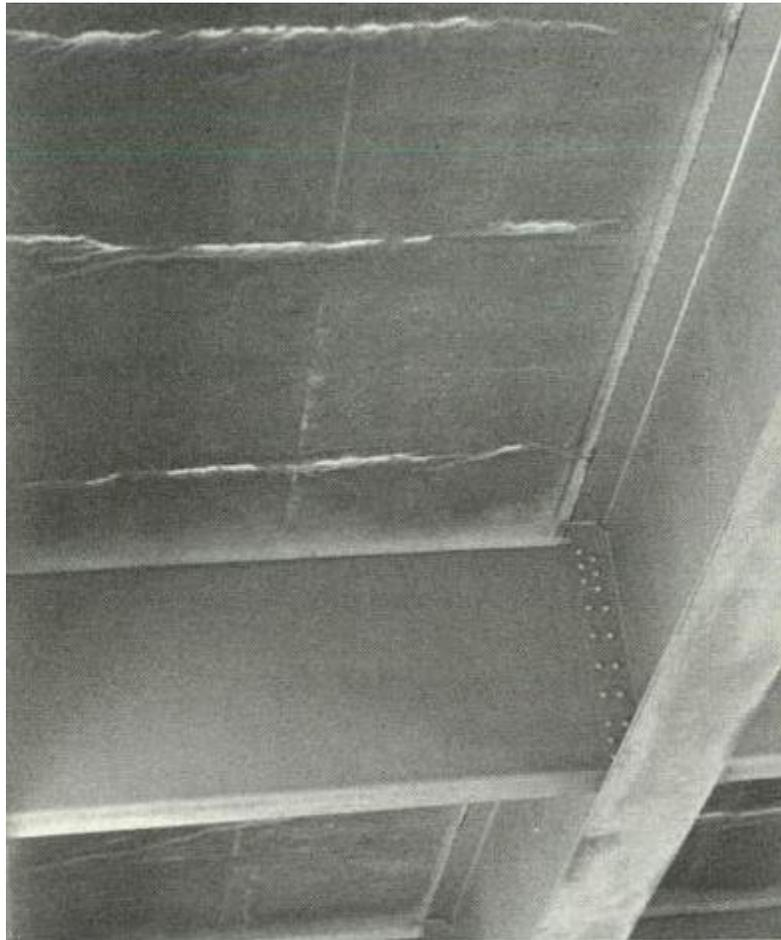
**Figure 2. 1 Representative deck cracking on the underside of a deck slab (Manning 1981).**
