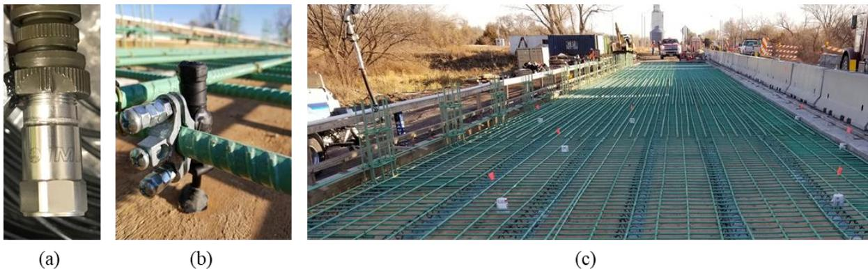
**Figure 4. 5 (a) PCB 603C01 sensor; (b) waterproofed sensor fixed to rebar; and, (c) protected sensors fixed to rebar for T3-BR2.**
