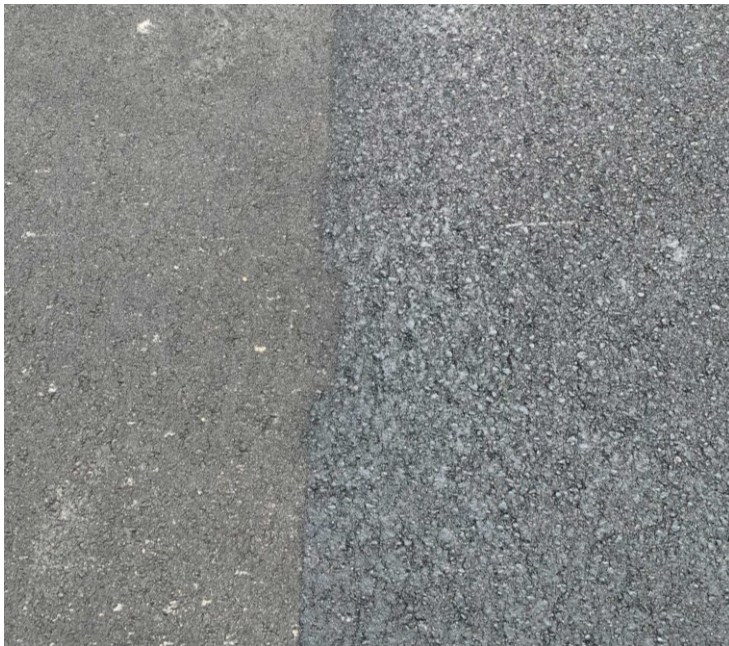
Figure 4 Pavement before (left) and after (right) the bio fog seal application
