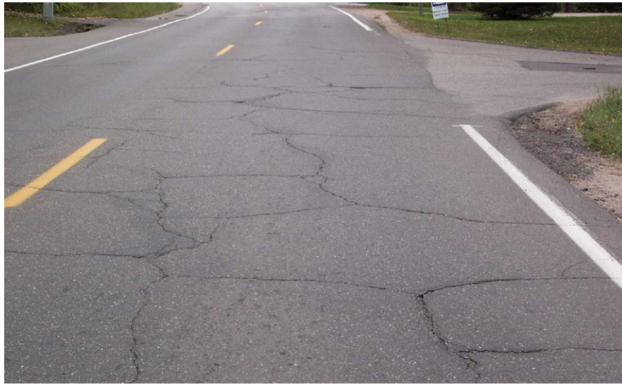
Figure A.9 Low Severity Multiple Cracking (MnDOT, 2011)
