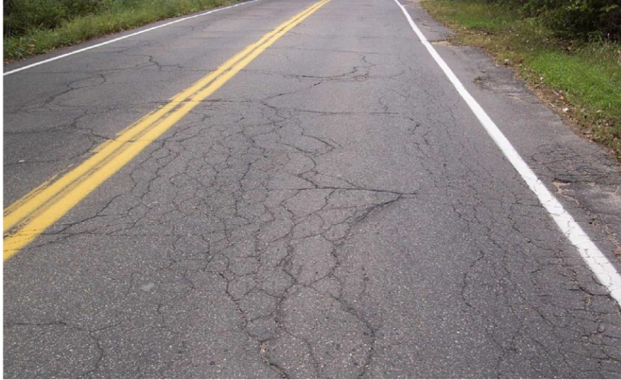
Figure A.13 Alligator/fatigue Cracking, Medium Severity (MnDOT, 2011)
