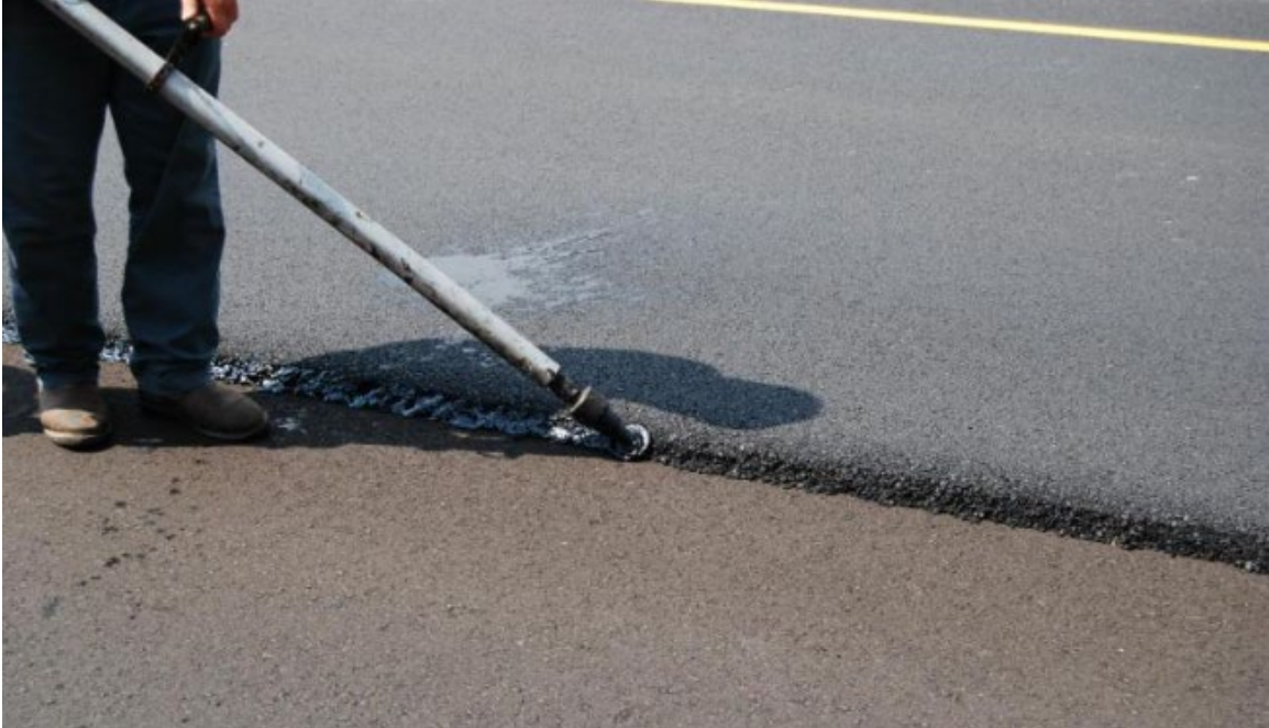
Figure 9. Joint adhesive application [36]
