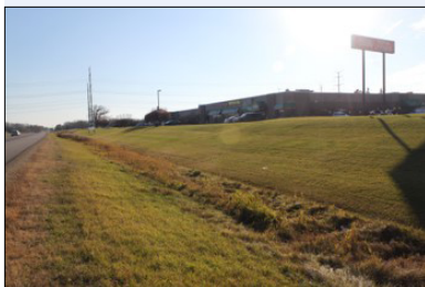
Swales in MnDOT's right of way can infiltrate stormwater runoff from roads.
