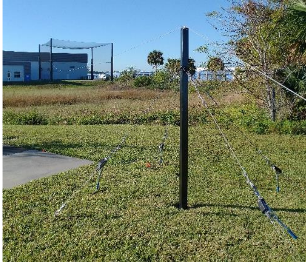
Figure 110. Support pole on large zipline
