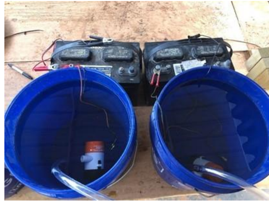
(b) bilge pump setup
