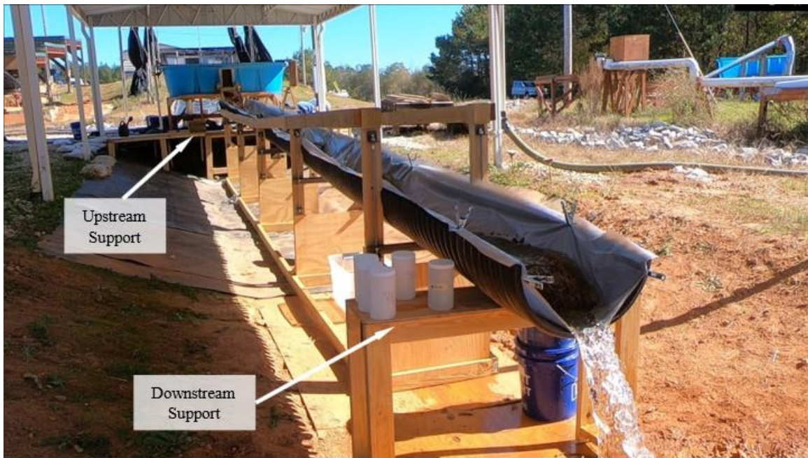
Figure 5-7: Post-construction Flume Setup
