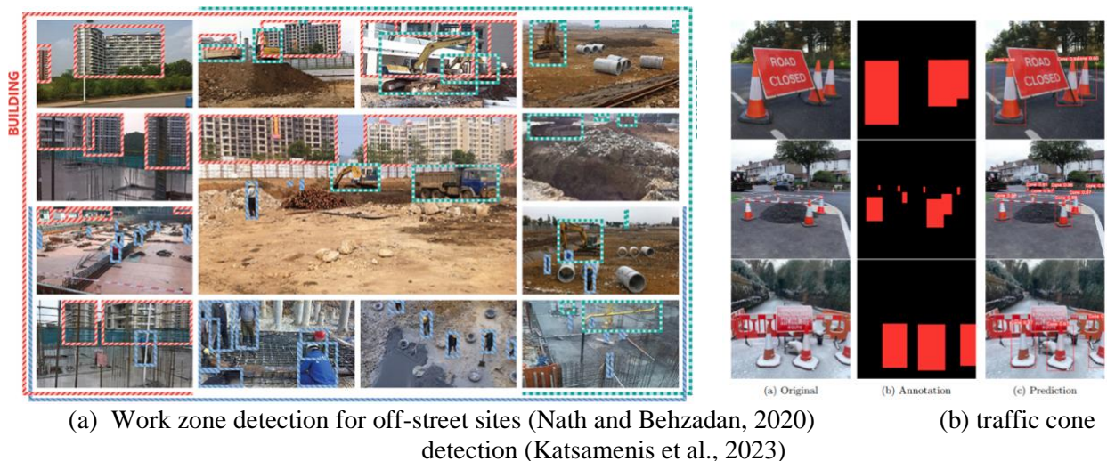
Figure 7. Examples of work zone detection research
