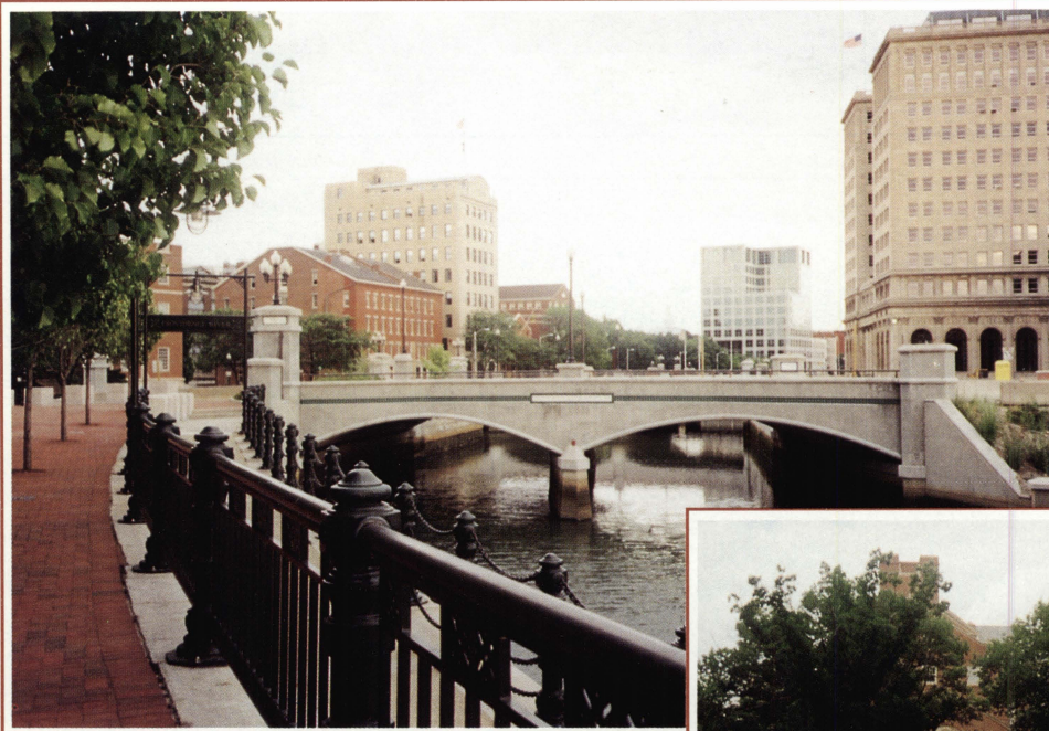
The newly constructed riverwalk and Memorial Avenue Bridge enhance the Woonasquatucket River.
