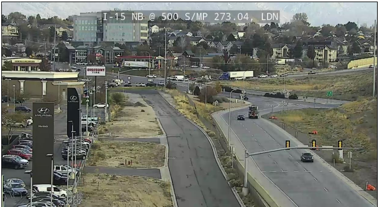
Figure 11: Sample Frame from Location 500 S - Northbound
