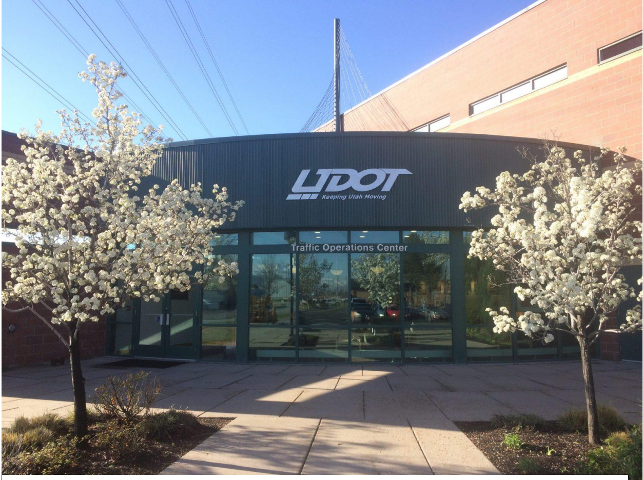
Figure 17: Utah Department of Transportation - Traffic Operations Center
