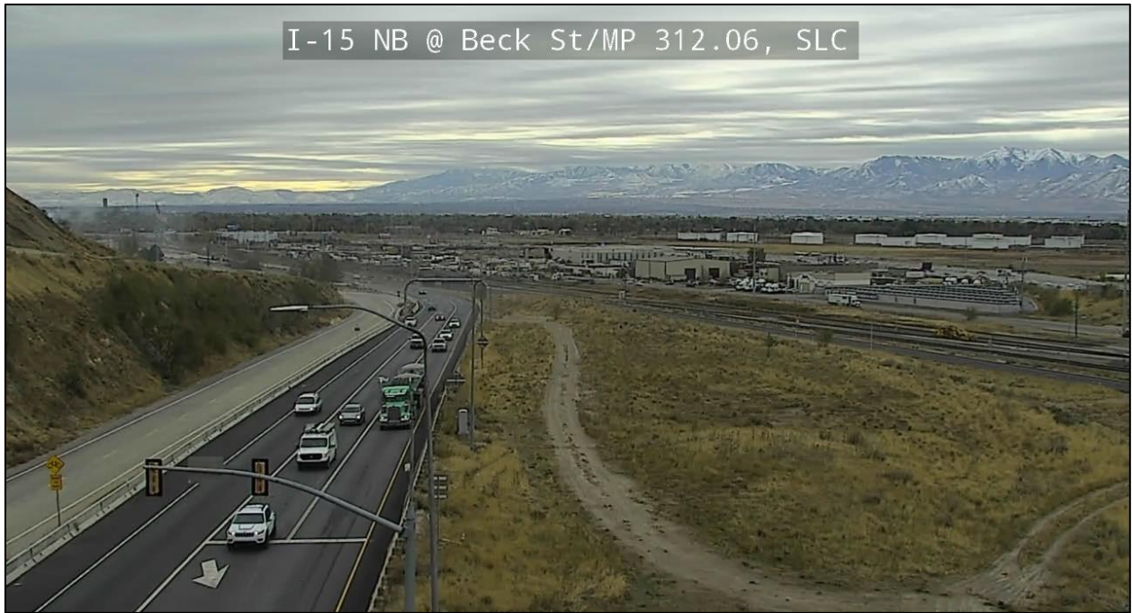
Figure 12: Sample Frame from Location Beck St - Northbound
