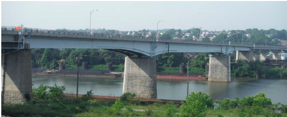
Fig. 3.5 – Photo of the Clairton-Glassport Bridge
