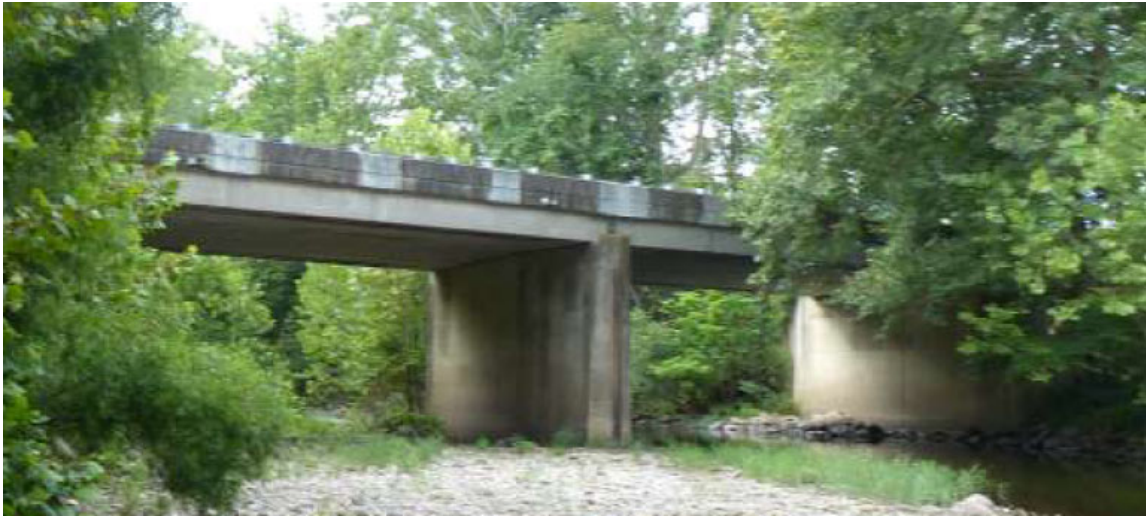
Fig. 3.6 – Photo of the Cooks Mill Bridge.
