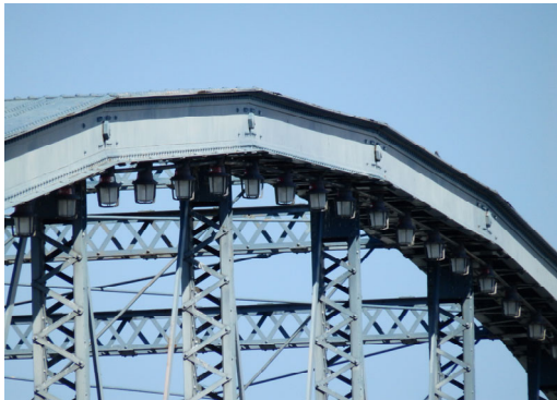
Fig. 5.2 – Close-up view of the center truss, with the top, diagonal, and bottom member. The west truss and some strain gages are also visible. Photos by Piervincenzo Rizzo.
