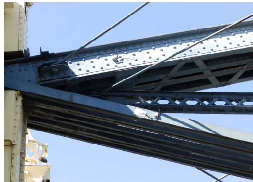
Fig. 5.2 – Close-up view of the center truss, with the top, diagonal, and bottom member. The west truss and some strain gages are also visible. Photos by Piervincenzo Rizzo.
