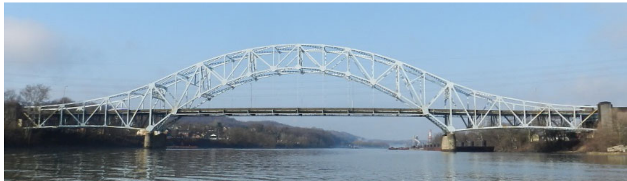
Fig. 3.1 – Location of the sensing system on the Elizabeth bridge (Elevation looking downstream). From left to right, piers 10, 11, 12, and 13 are visible.
