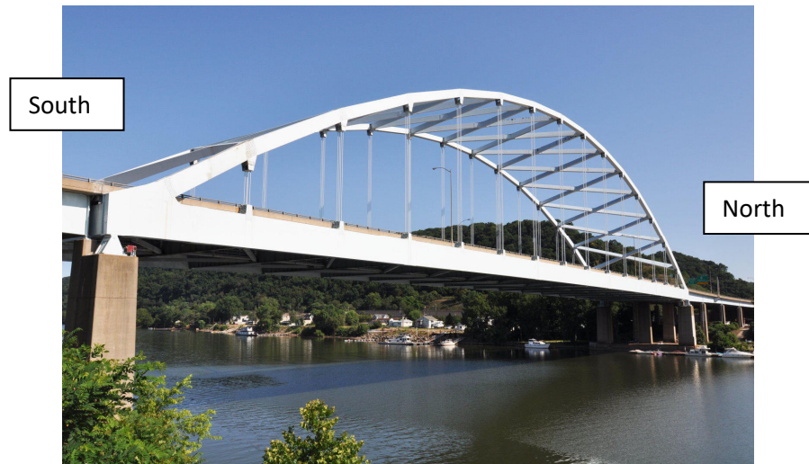
Fig. 3.2 – The Neville Island bridge. Source: https://www.penndot.gov/RegionalOffices/district-11/PublicMeetings/Documents/SR0079%20A61%20Detour%20Slides%201-21-2020.pdf
