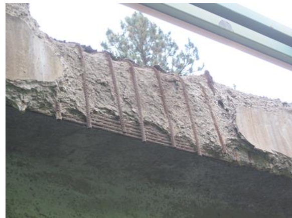
(f) Midspan Close-up View of Selected 50-ft (15.24-m) Long Girder
