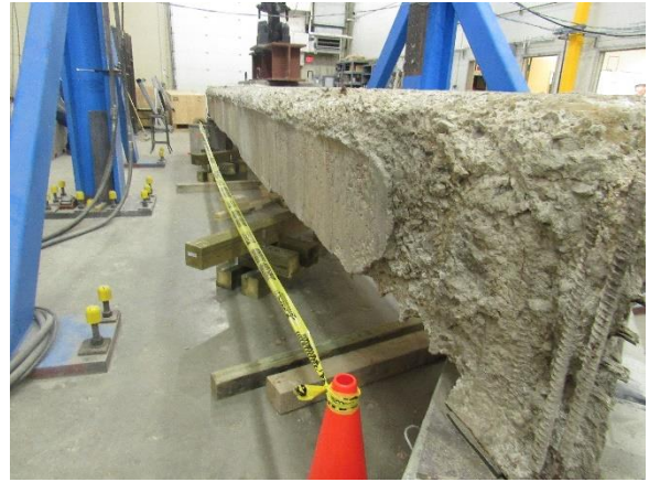
(b) Stem Cover Deterioration
