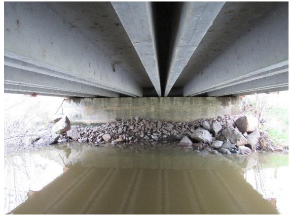
(b) Underneath of bridge
