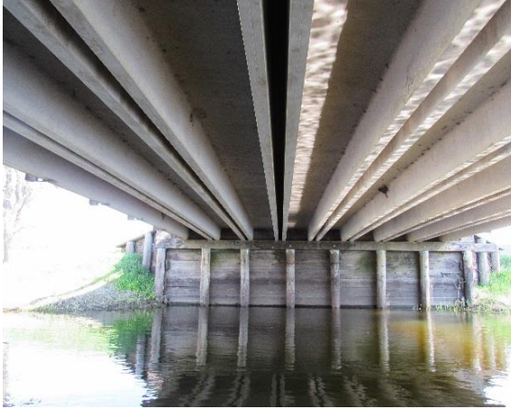
(a) Underneath of Bridge
