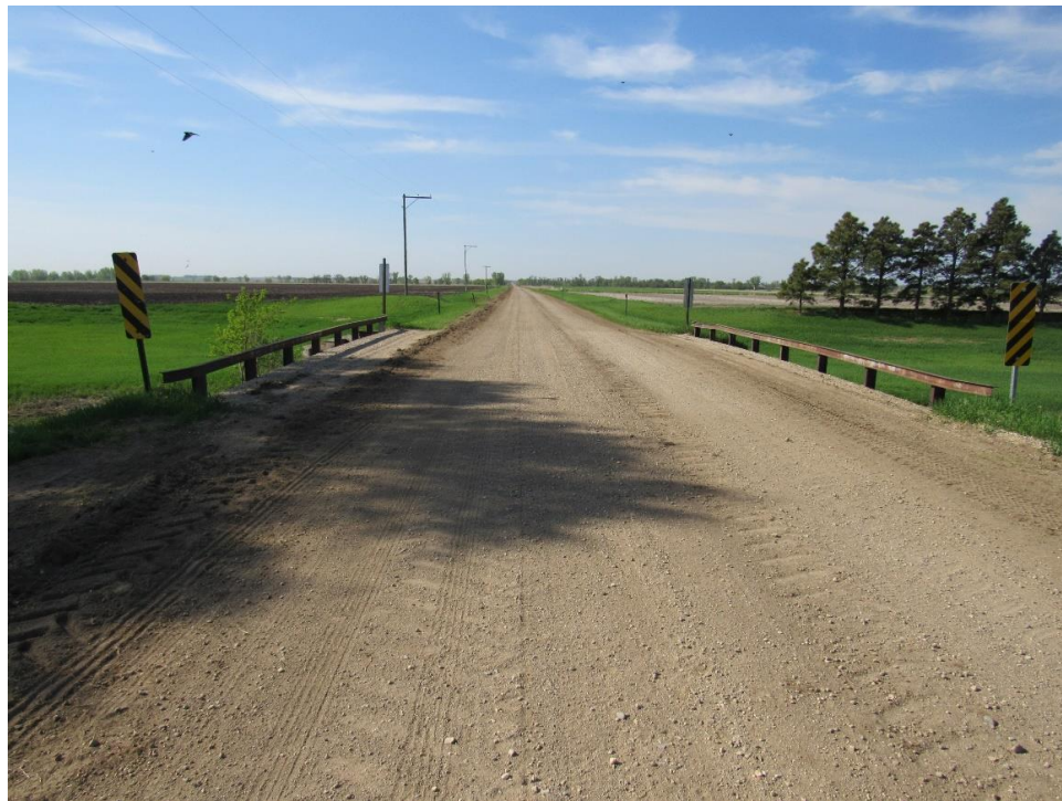
(b) Alignment Facing South
