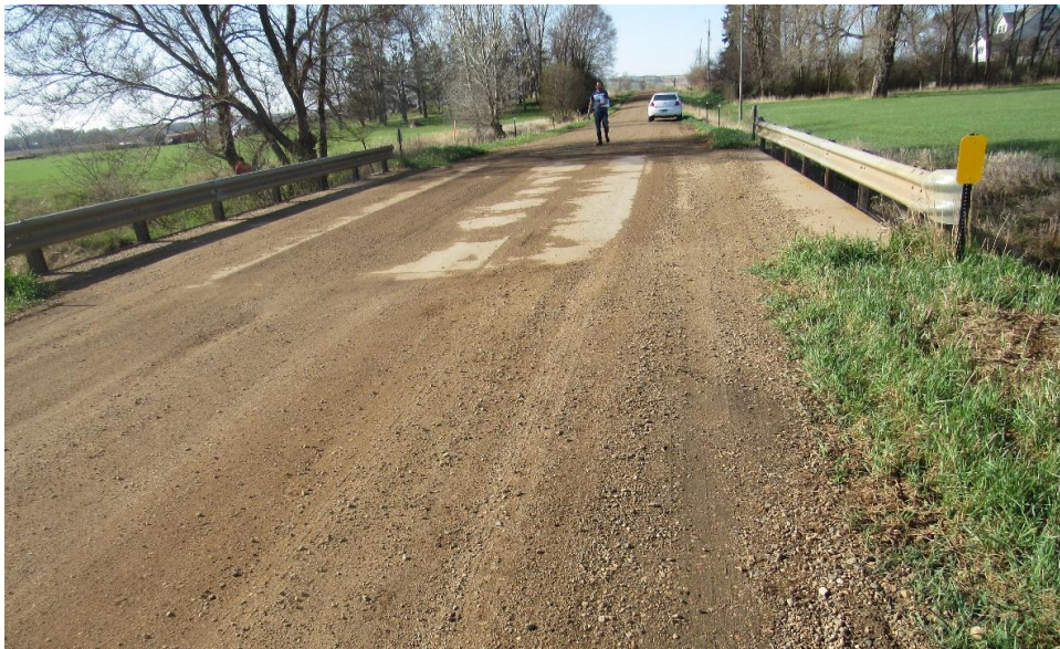
(b) Alignment Facing South
