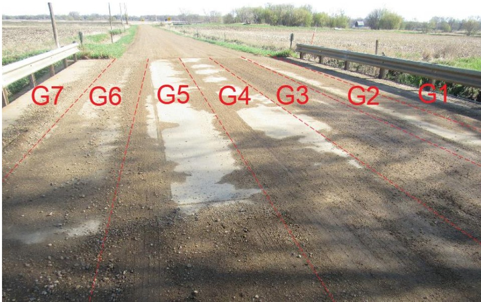
(a) Alignment Facing North
