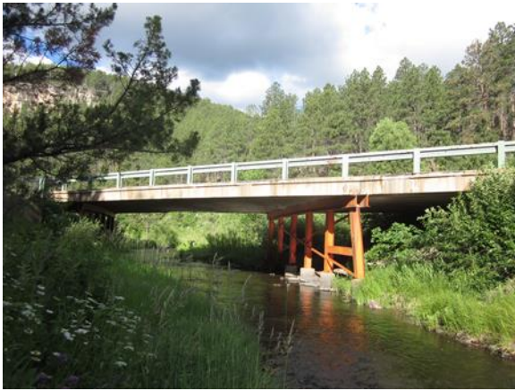
(a) Bridge 52-313-265 (Nemo Road)
