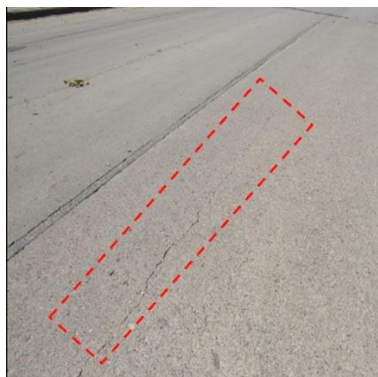
(j) Flange Cracking (CS-2)
