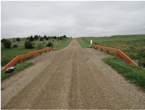
(a) Top view of bridge
