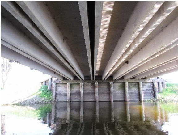
(c) Underneath of bridge
