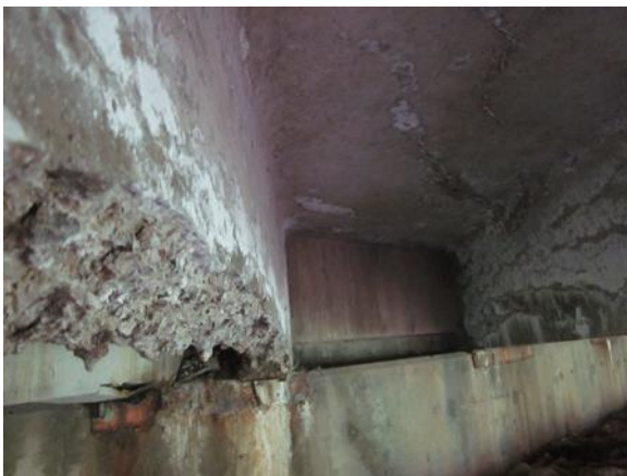
(c) Selected 30-ft (9.14-m) Long Girder – Underneath View
