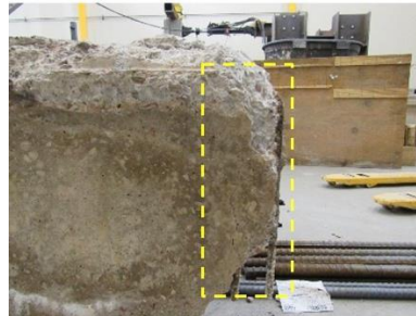
(t) Stem Exposure of Transverse Rebar (CS-2)
