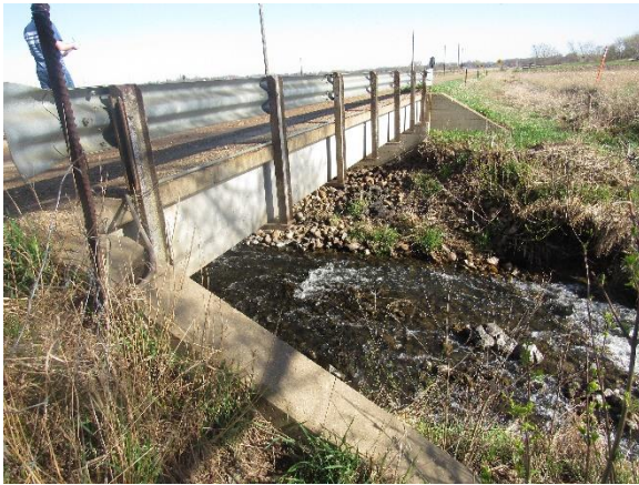
(a) Side view of bridge
