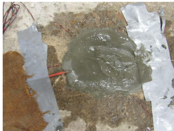
(b) After Pouring Grout
