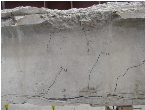
(a) First Flexural Crack at Midspan
