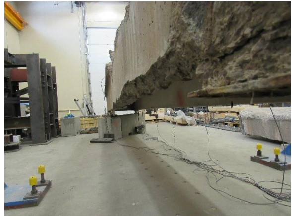
(b) Stem Cover Deterioration for 50-ft (15.24-m) Girder
