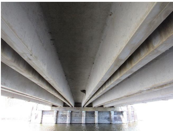
(c) Underneath of bridge
