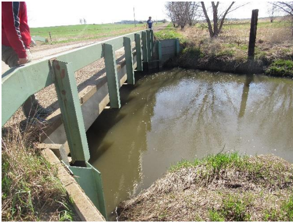
(a) Side view of bridge
