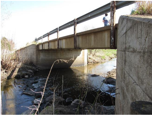
(a) Side view of bridge
