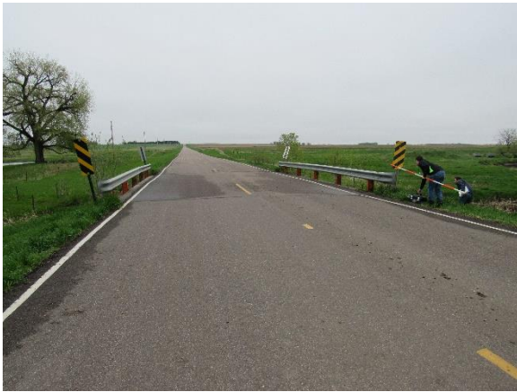
(a) Top view of bridge
