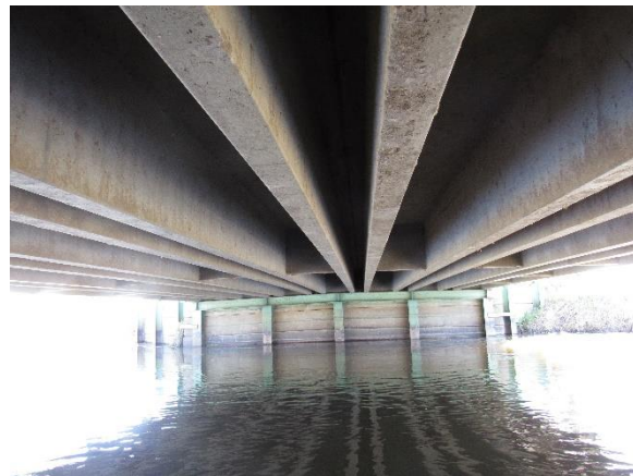
(f) Underneath of bridge
