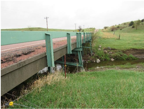
(a) Side view of bridge
