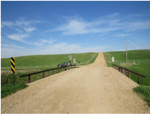
(a) Top view of bridge
