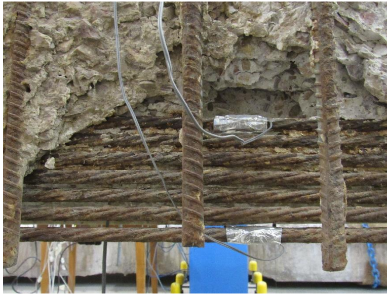
Figure 8.11 – Installation of Steel Tendon Strain Gauges
