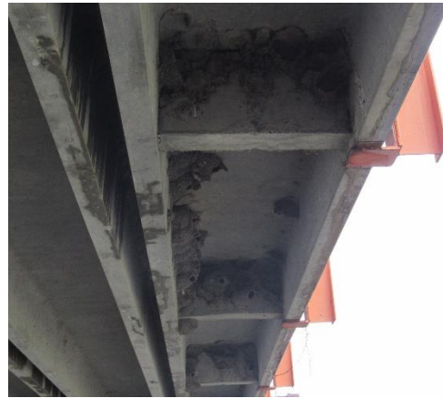
(b) Diaphragm at the exterior girder
