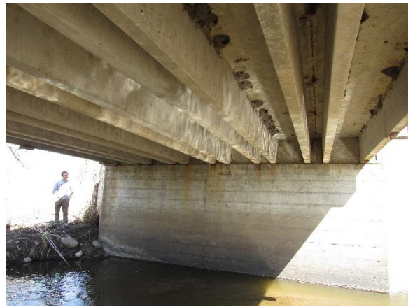
(f) Underneath of bridge
