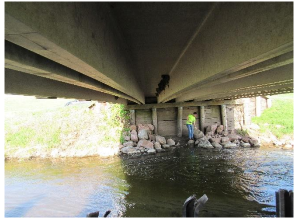
(b) Underneath of bridge
