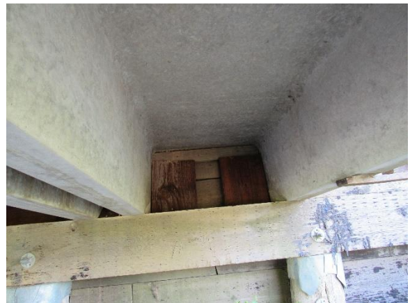
(f) Wooden diaphragm at end of girder
