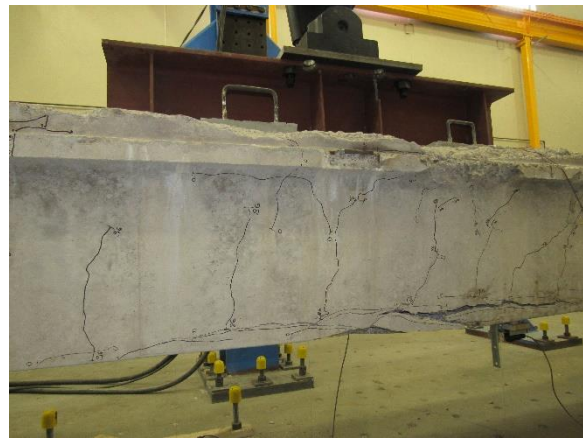
(b) Extension of Flexural cracks
