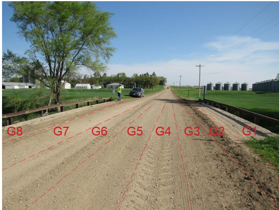
(a) Alignment Facing North
