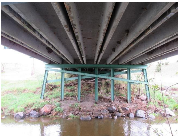
(c) Underneath of bridge
