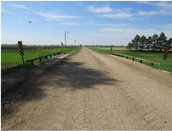
(a) Top view of bridge
