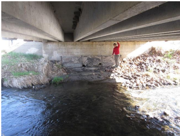
(e) Underneath of Bridge
