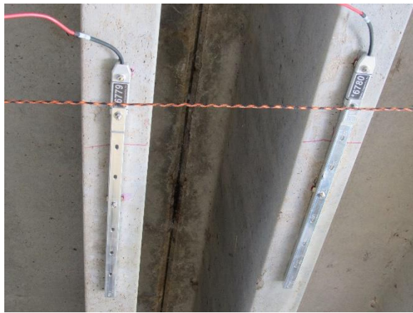
(a) Installation of Strain Gauges with Extension
