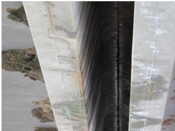
(e) Efflorescence
