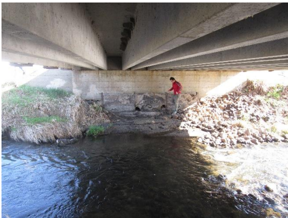
(e) Underneath of bridge
