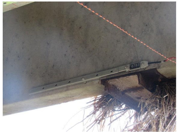
(b) Strain Gauges at Side due to Railing
