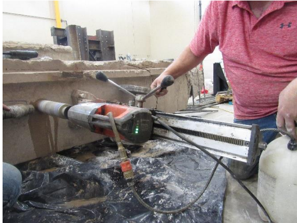
(a) Coring at Stem of 50-ft Long Girder
