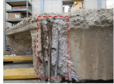
(u) Stem Exposure of Transvers Rebar (CS-3)
