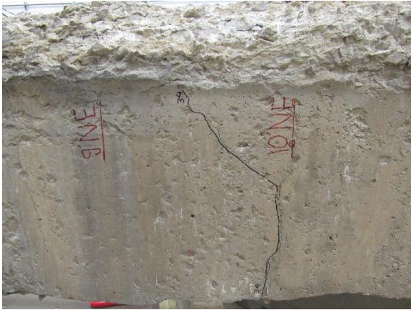
(a) First Shear Crack at North End
