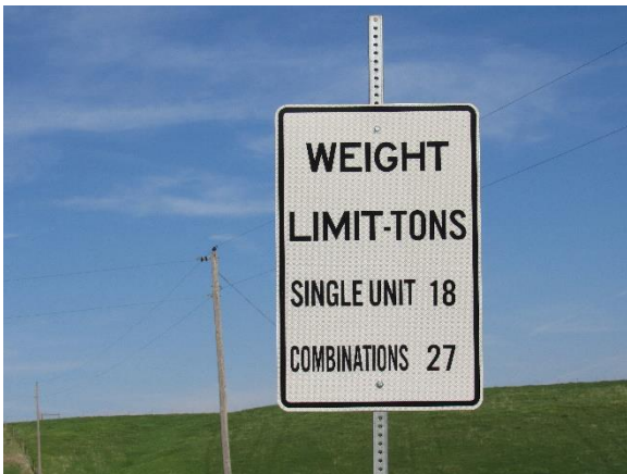
(e) Posting of bridge
