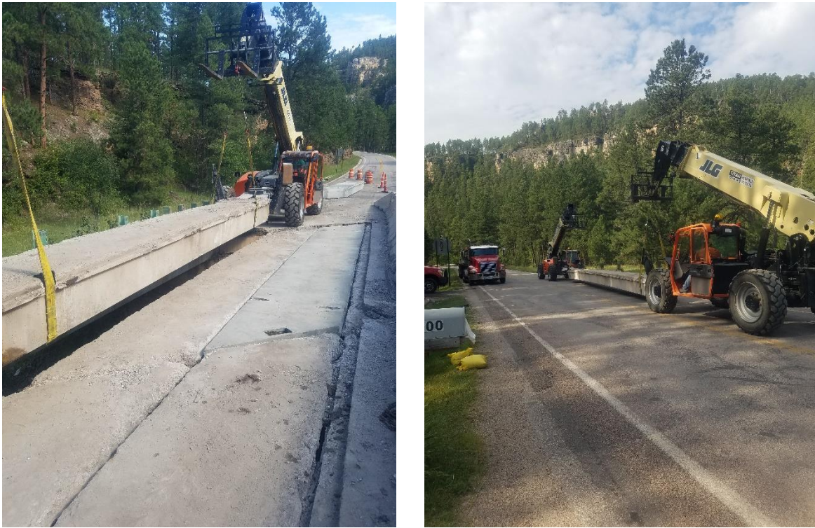
Figure 8.3 – Extraction and Transportation of Salvaged Double-Tee Girders
