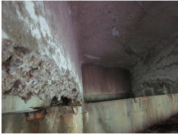
(a) Underneath View of Girder
