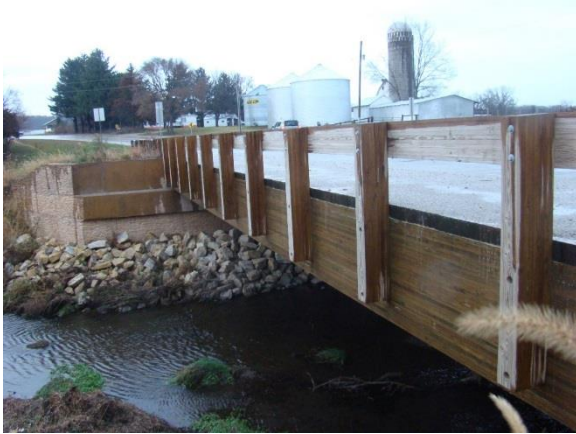
Figure A.16: Timber Railing for Timber Bridges
