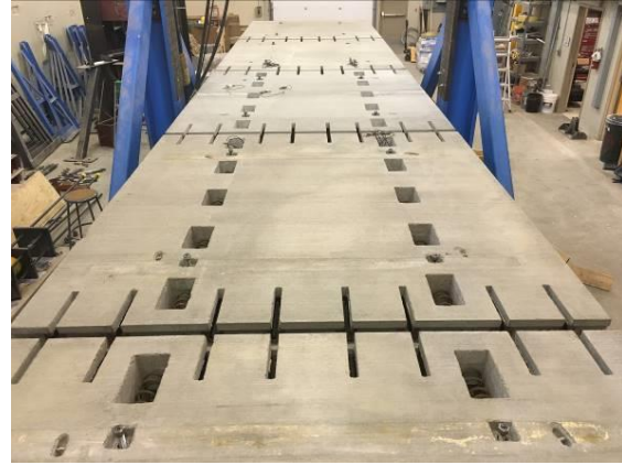
Figure 6.10: Installation for Full-depth Deck Panels on Precast Girders
