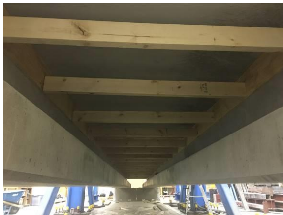
Figure 7.4: Grouted Haunch Region Formwork Installed between Girders
