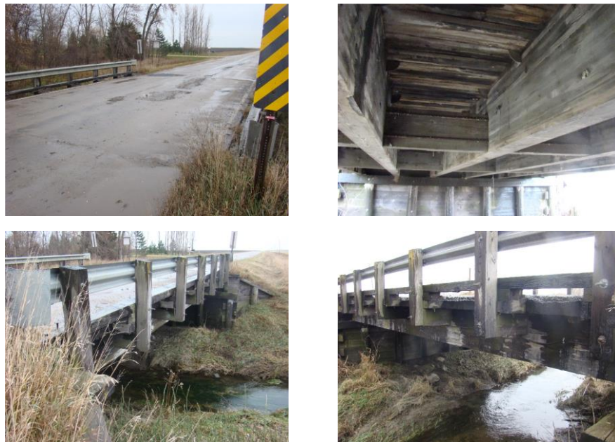
Figure 5.28: Glulam Timber Bridge No. 9967 in Faribault County, Minnesota
