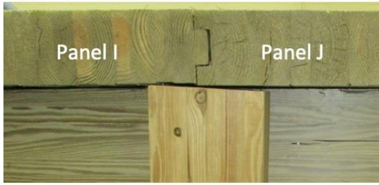
(b) Panel I-to-J Connection (East Side) at 0 Cycles
