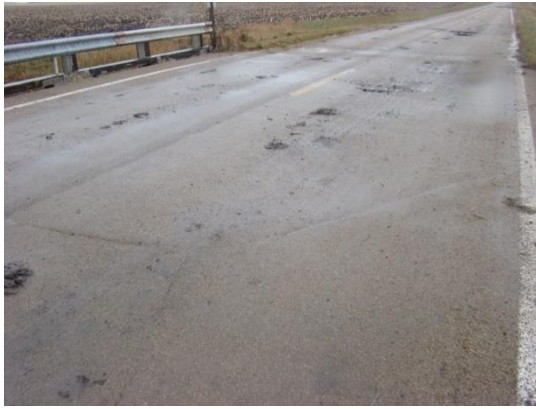
(a) Asphalt Overlay
