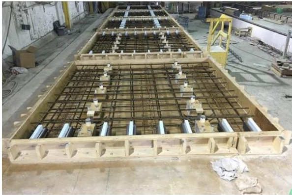
(a) Panel Formwork
