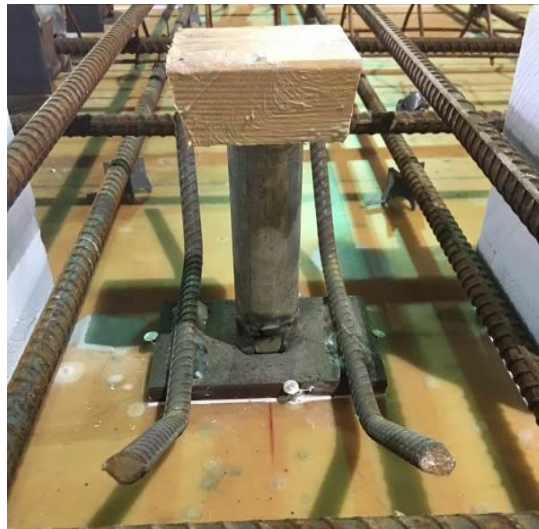
Figure 7.3: Leveling Bolt Construction Detail
