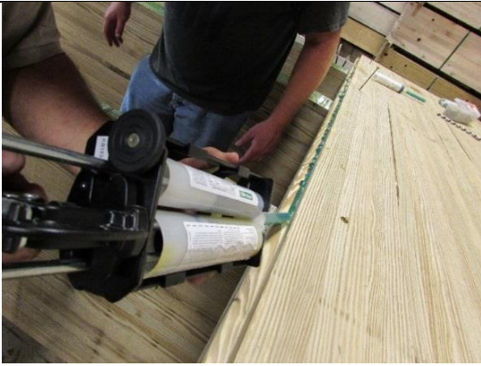
(b) Placement of Epoxy between Girder and Deck
