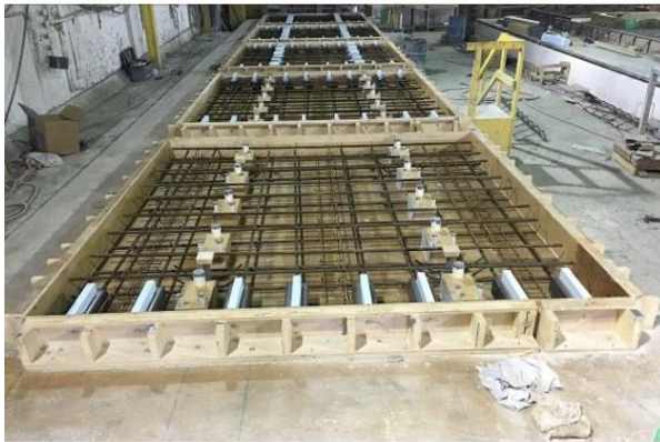
(a) Panel Formwork
