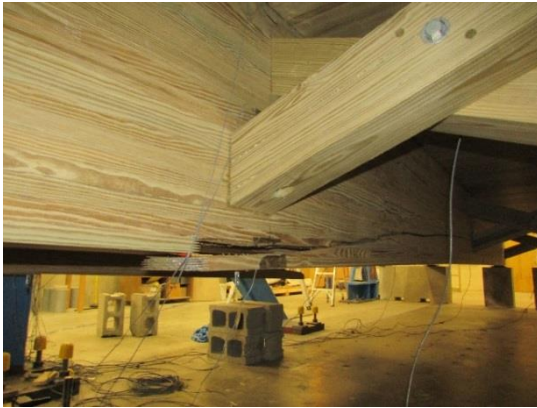
(c) Failure of Interior Girder
