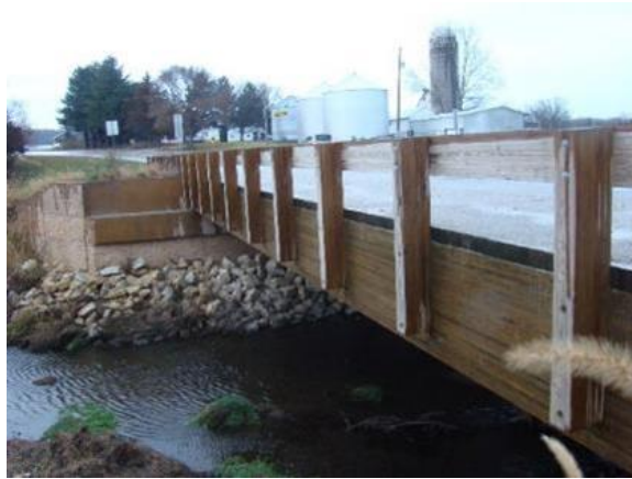
Figure 5.16: Glulam Timber Bridge in Buchanan County, Iowa
