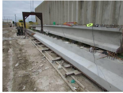
(b) Formwork Removal
