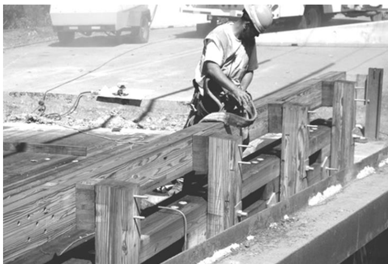
Figure 5.30: Railing on a Glulam Bridge (after laminatedconcepts.com)
