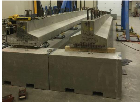
(b) Girder Placement on Abutments
