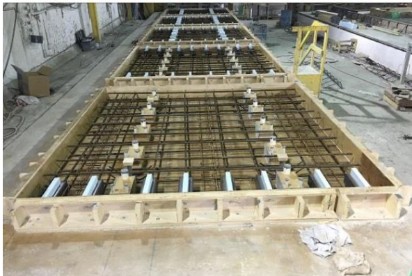
(a) Panel Formwork
