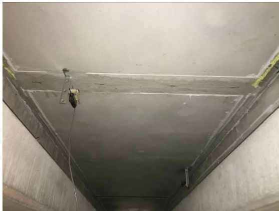
(a) Joint with Non-Shrink Grout – Deck Underneath
