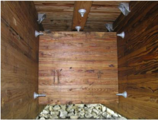
(a) Solid Glulam Diaphragm (after Hosteng, 2013)
