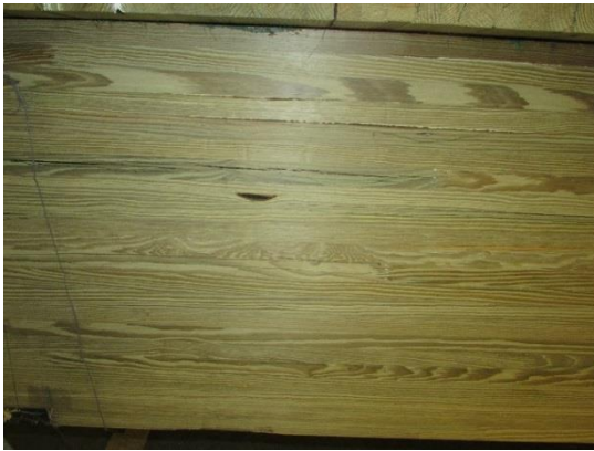
(e) Condition of East Girder at Mid-span
