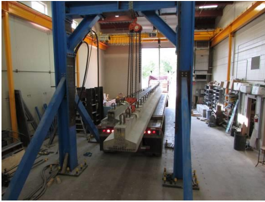
(a) Girder Unloading
