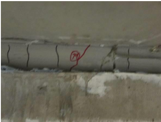
(a) 16-ft North of Mid-span (Girder B)
