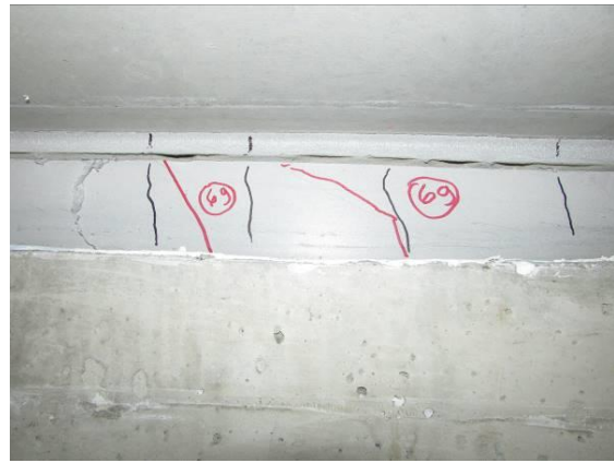
(b) 14-ft South of Mid-span (Girder A)
