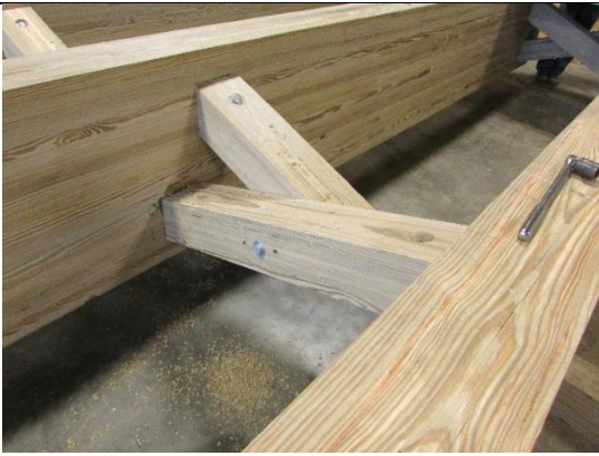
(a) Installation of Cross Braces
