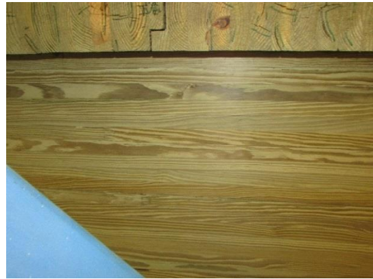
(f) Condition of East Girder at Mid-span
