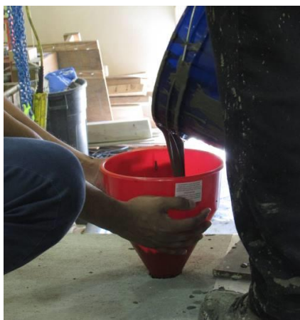
(a) Pouring in Hidden Pockets
