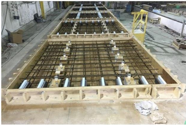
(a) Panel Formwork
