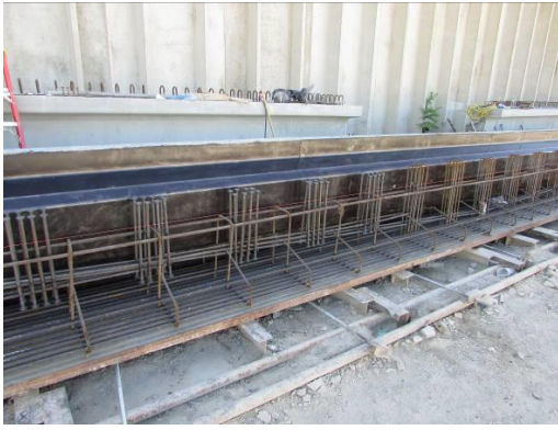
(a) Placement of Bars and Prestressing Strands
