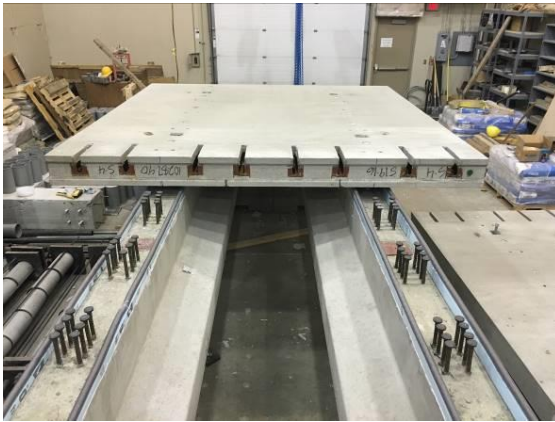
Figure 6.10: Installation for Full-depth Deck Panels on Precast Girders
