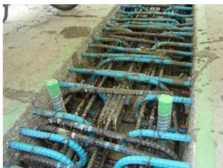
(a) Photograph of Longitudinal Joint
