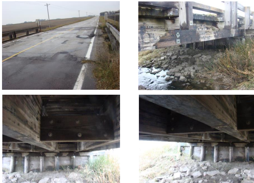
Figure 5.27: Glulam Timber Bridge No. 22519 in Faribault County, Minnesota
