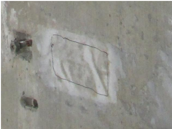
(a) Non-Shrink Grout at 125,000 Cycle
