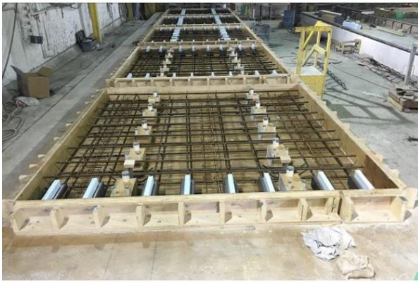
(a) Panel Formwork
