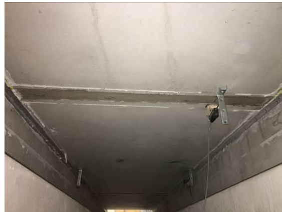
(b) Joint Latex Modified Concrete – Deck Underneath
