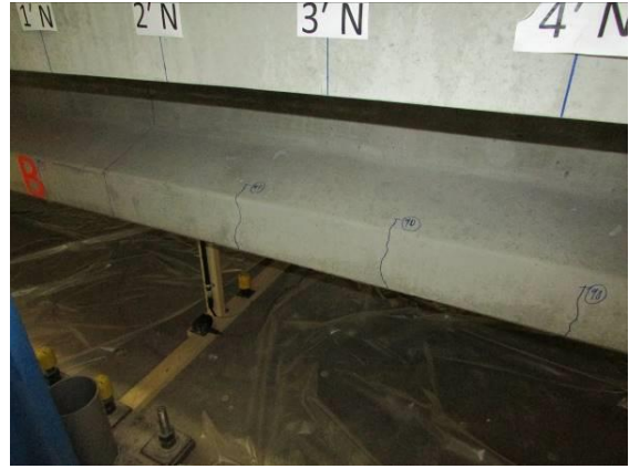
(b) First Crack, Mid-span of Girder B at P = 251 kips
