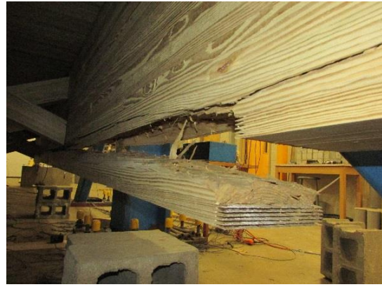
(b) Failure of West Girder
