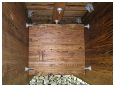
(a) Solid Glulam Diaphragm, (after Hosteng, 2013)
