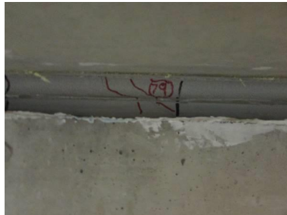
(b) 14-ft South of Mid-span (Girder B)
