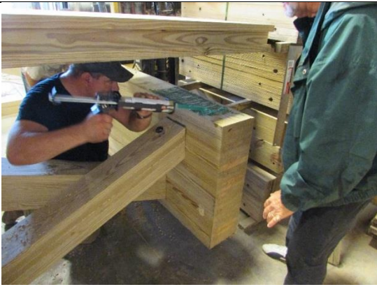
(b) Placement of Epoxy between Girder and Deck
