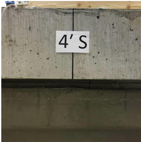
(a) Observed Crack at 25,000-Load Cycle
