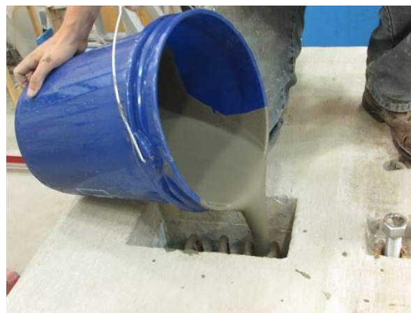
(b) Pouring in Open Pockets
