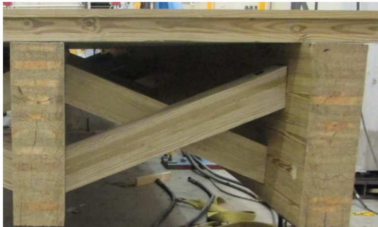
Figure 5.20: Glulam Cross Braces for Girder Timber Bridges
