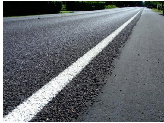
(b) Asphalt Chip Seal (after Gruen-Wald 2011)
