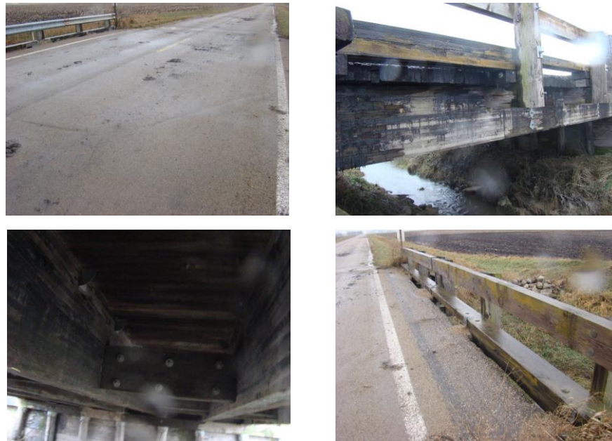
Figure 5.24: Glulam Timber Bridge No. 22508 in Faribault County, Minnesota
