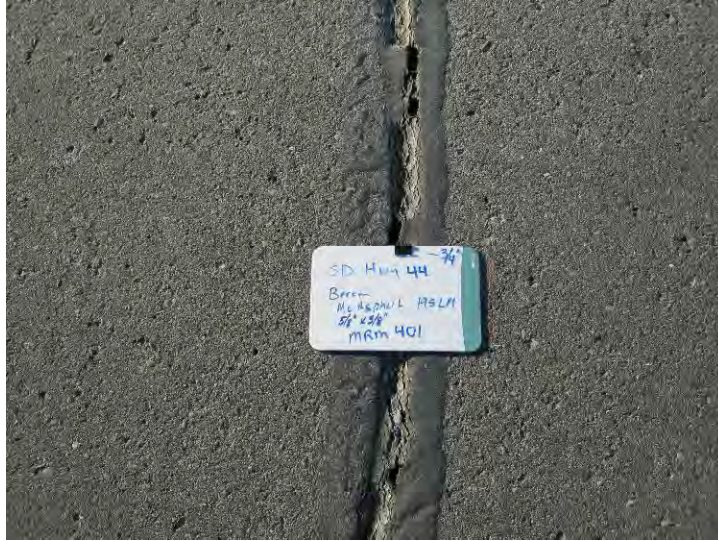
Figure 11: Crack sealant on Highway 44, MRM 401 – winter 2013.
