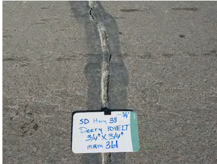
Figure 9: Crack sealant on Highway 38, MRM 361 – winter 2013.
