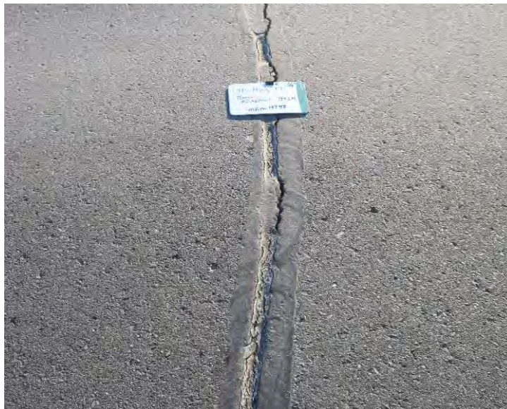
Figure 8 Crack sealant on Highway 17, MRM 47.48 – winter 2013.
