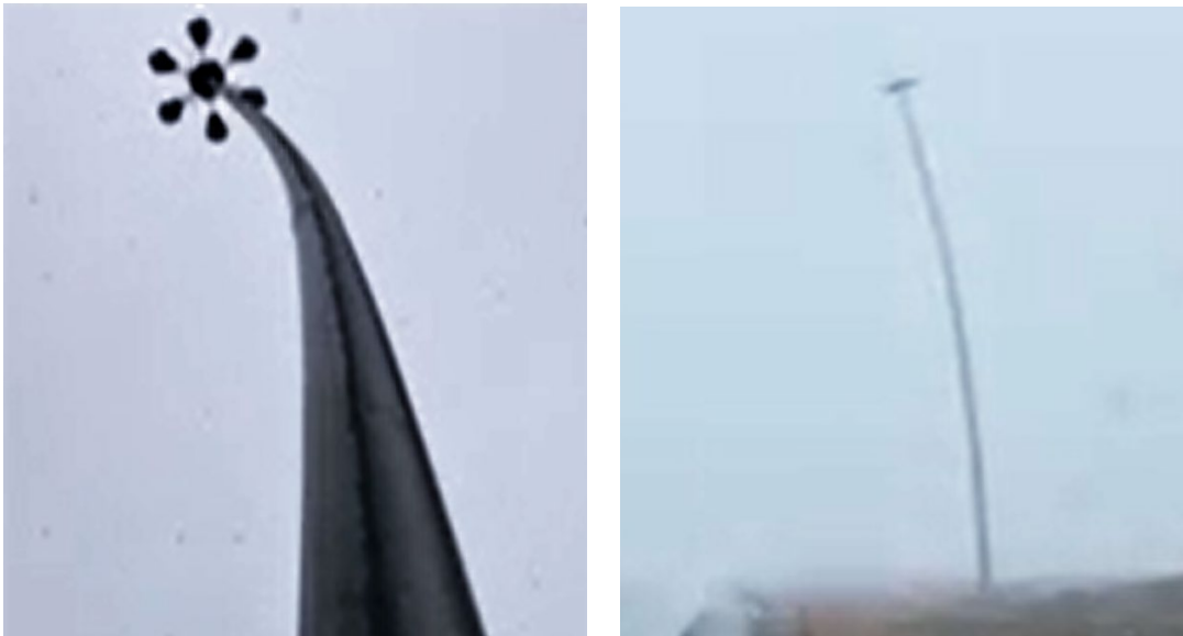
Figure 31. Images from cell phone footage showing deflection of two poles
