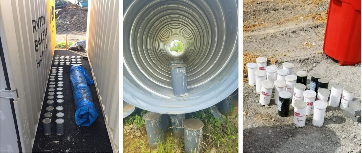
Figure 1-4: Improper jobsite curing of cylinders that neither meet ALDOT 501 nor AASHTO T23 requirements (Source: NRMCA)
