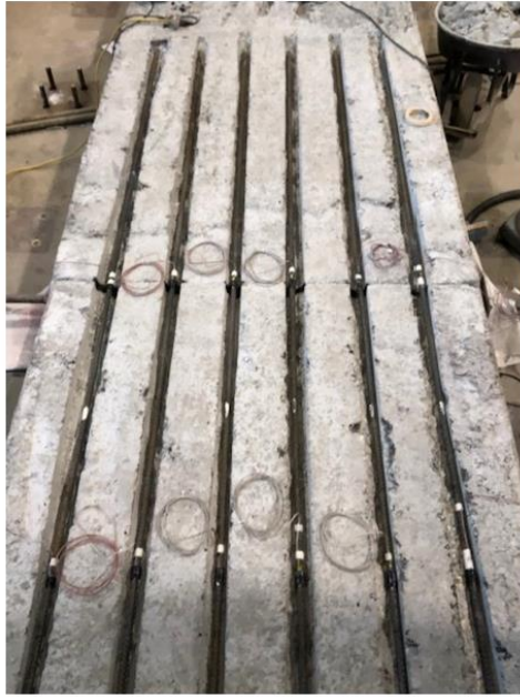
Figure 3.18 Placement of #6 Bars and Strain Gauges
