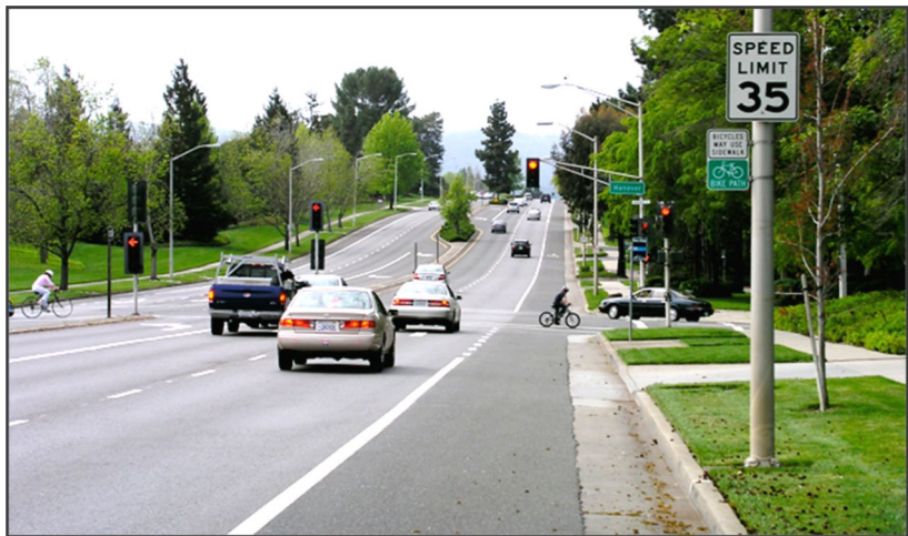
Figure 1-3: Other Principal Arterial in California
