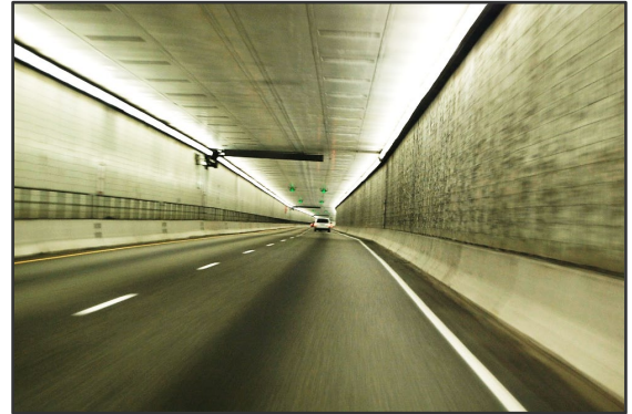
Figure 2-2: View from Inside the Eisenhower Tunnel
