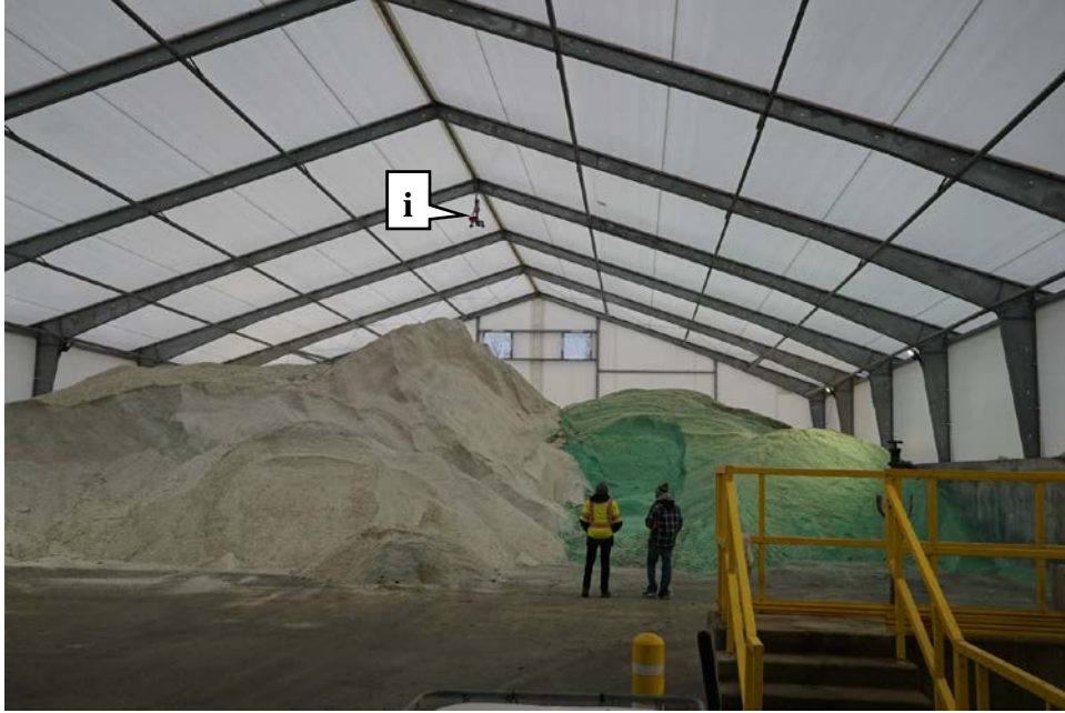
(a) Lebanon Unit Permanent Install
