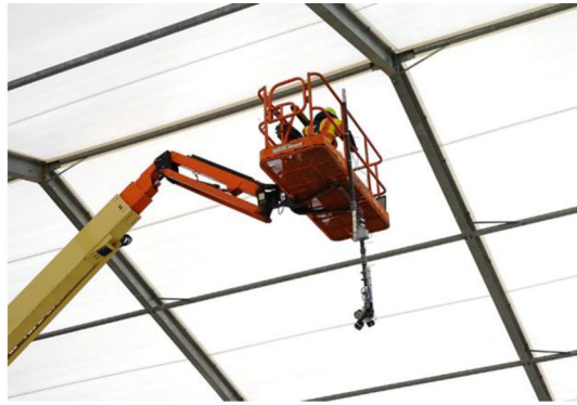
(a) Installation and Data Collection on Boom Lift
