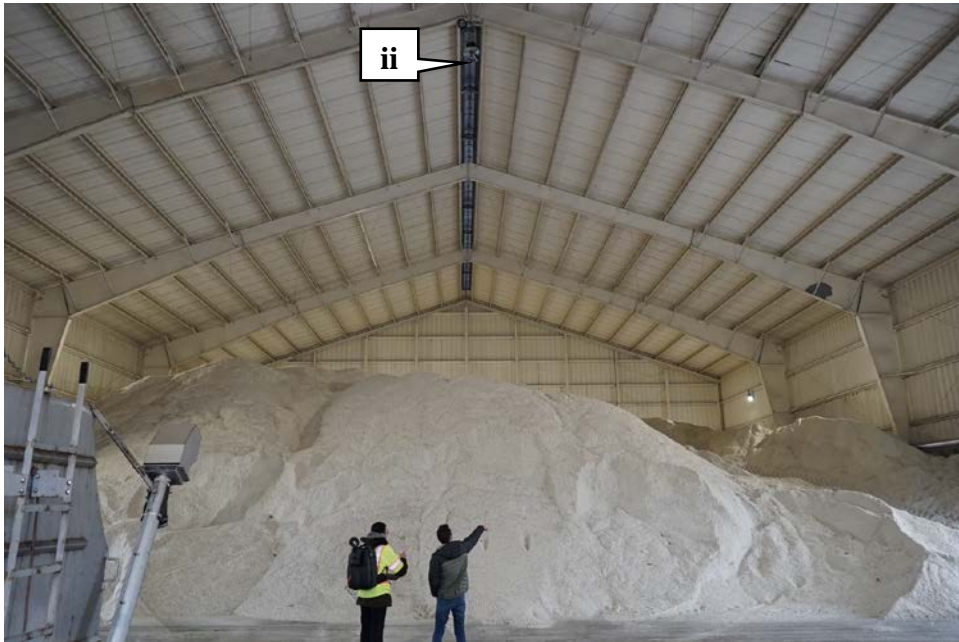
(b) Indianapolis Subdistrict Permanent Install
