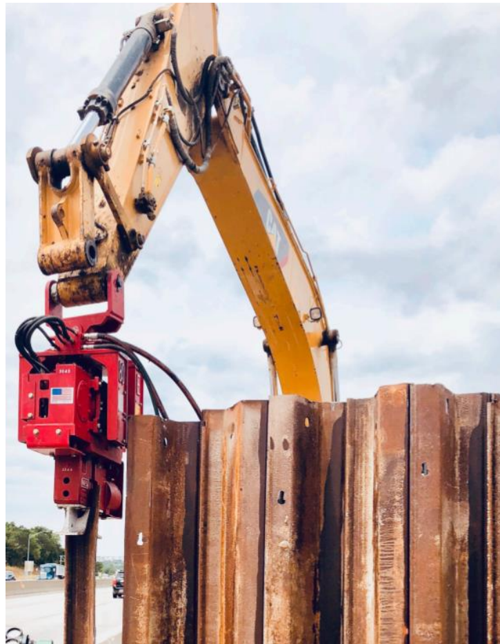
Figure B1. Excavator mounted vibratory hammer.
