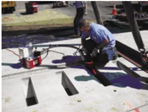
Demonstration of the precast post-tensioned concrete pavement system in Sikeston, Missouri.
