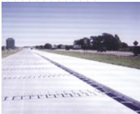
Construction of an unbonded concrete overlay on concrete pavement, I-44, Missouri.
