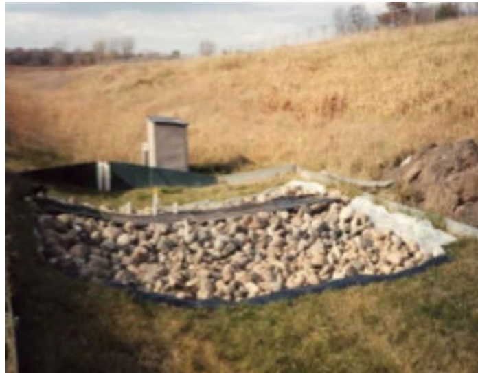
Figure E5. Pollution control research showing the check dam at MnROAD (Worel, 2021).
