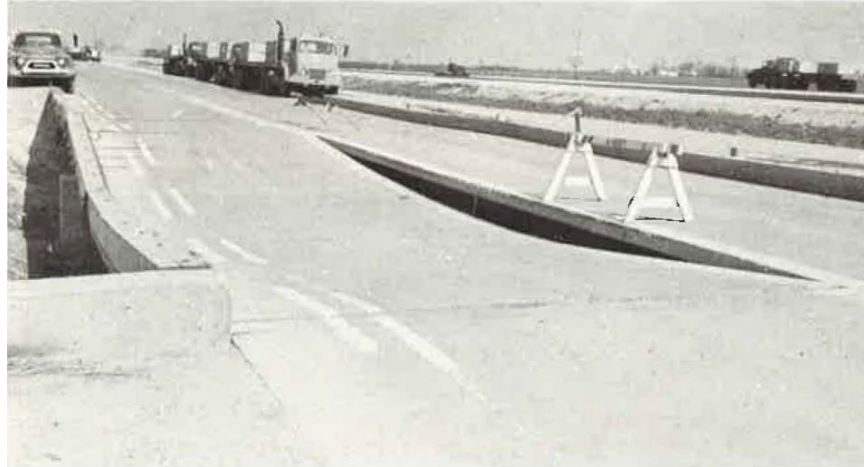
Figure E2. Bridge Testing at AASHO Road Test (Highway Research Board, 1962).
