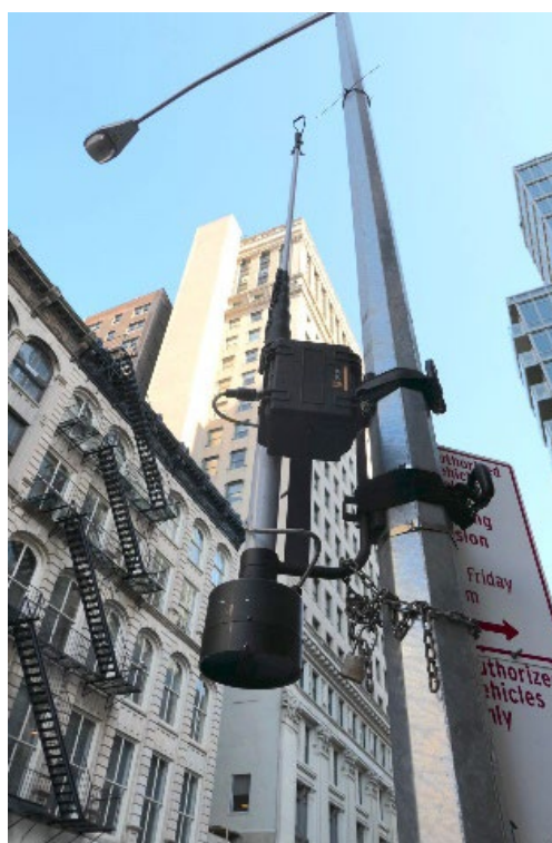
Figure 2-5: Miovision Scout Camera and Mounting Unit
