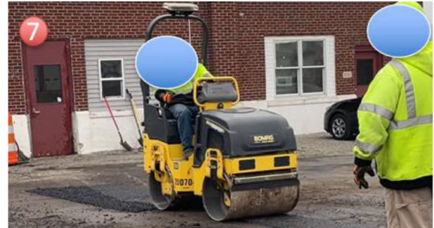
Figure 7.19 Shoveling asphalts–step seven.
