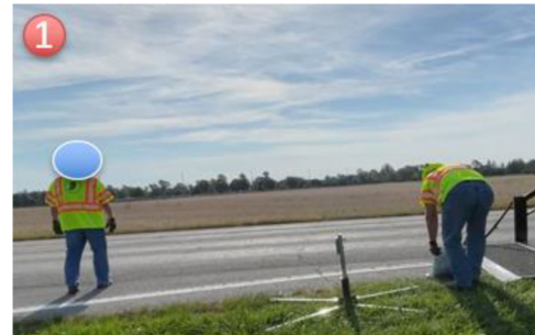
Figure 7.20 Pulling deer step one–dragging from the road to the curb.
