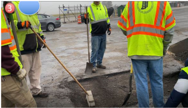
Figure 7.15 Shoveling asphalts–step three.
