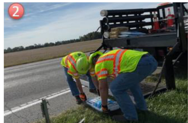
Figure 7.21 Pulling deer step two–dragging from the curb to the liftgate.
