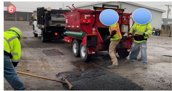
Figure 7.18 Shoveling asphalts–step six.
