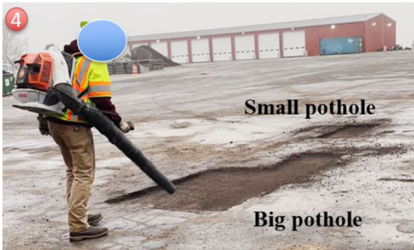
Figure 7.16 Shoveling asphalts–step four.
