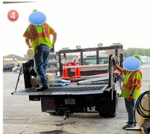
Figure 7.4 Lifting bags of dry concrete mix—step four.
