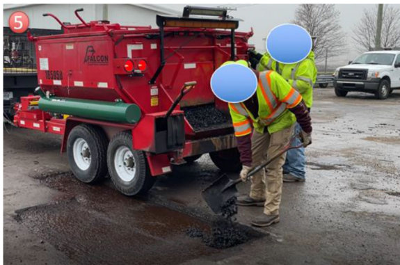
Figure 7.17 Shoveling asphalts–step five.
