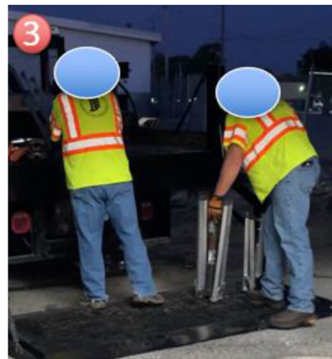
Figure 7.9 Lifting sign stands—step three.
