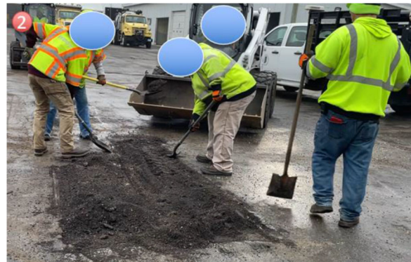
Figure 7.14 Shoveling asphalts–step two.
