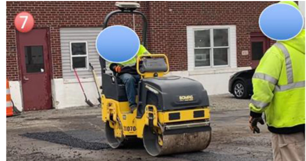
Figure 7.19 Shoveling asphalts–step seven.
