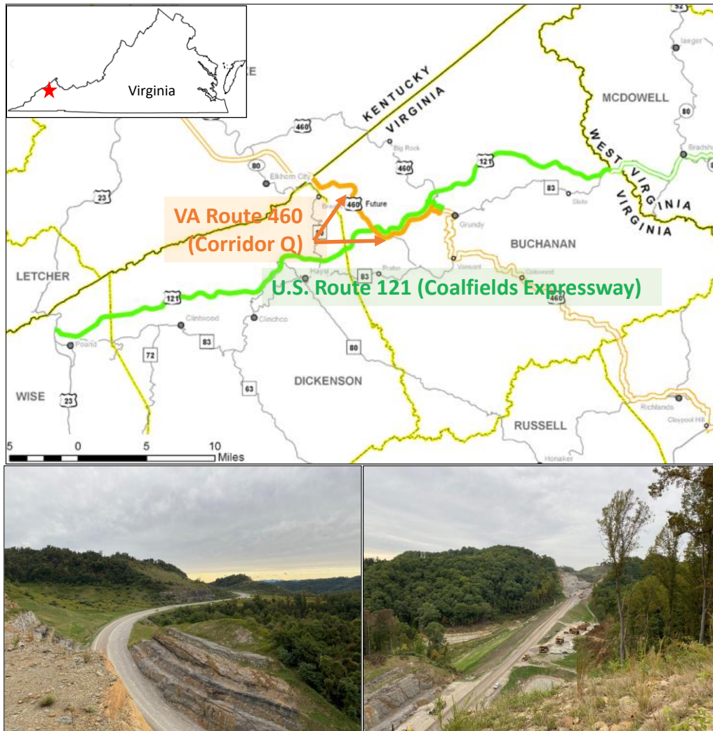
Figure 1. Virginia Route 460 / Corridor Q (top), and Corridor Q Under Construction (bottom)
