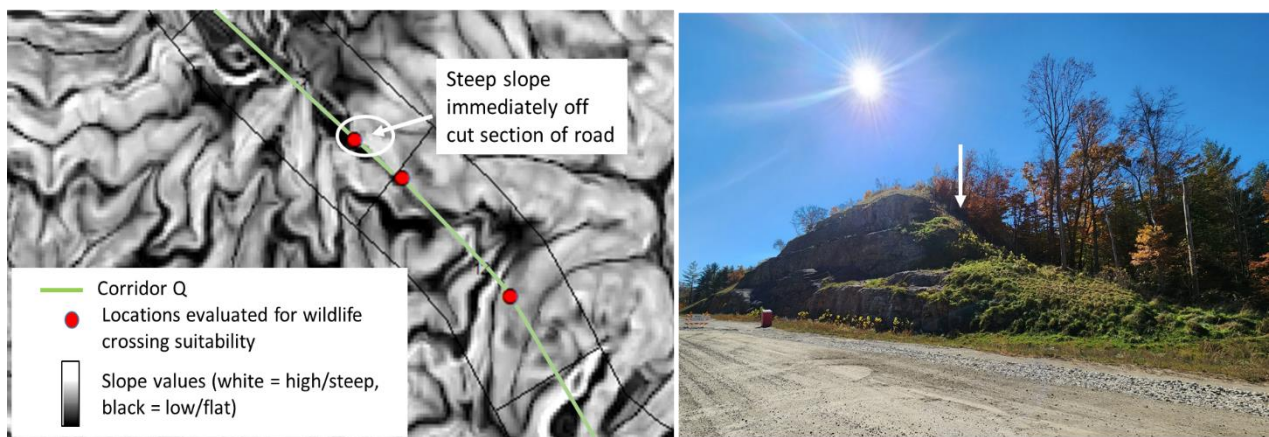
Figure 12. Illustrations of a Steep Slope Adjacent to a Cut Section of Road That Could Decrease the Likelihood of Elk Accessing an Overpass
