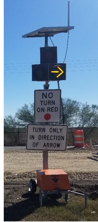
b. Flashing Proceed Indication.
