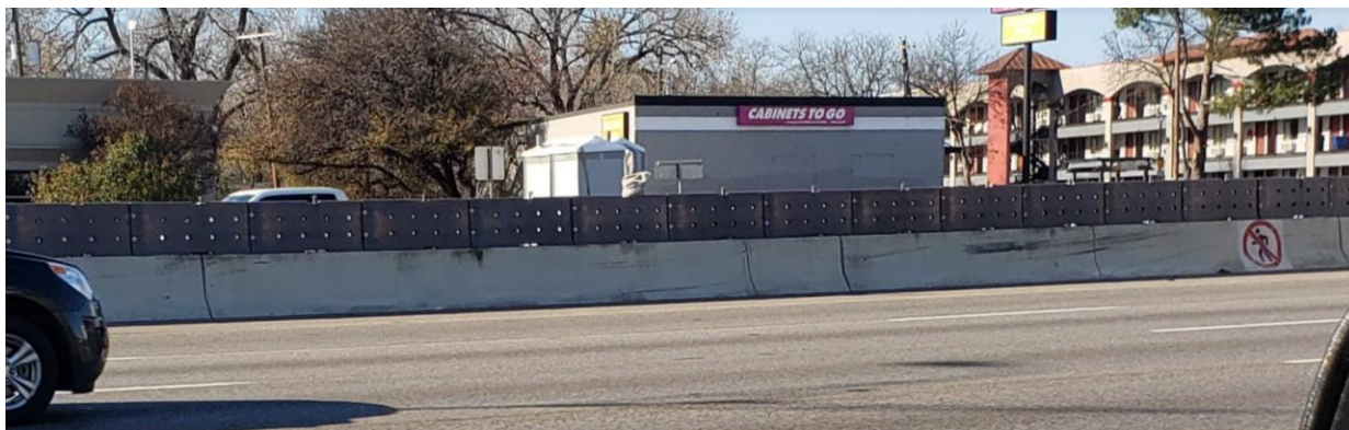
Figure 33. Stencil and Barrier on Top of Center Median on IH 35 in Austin.
